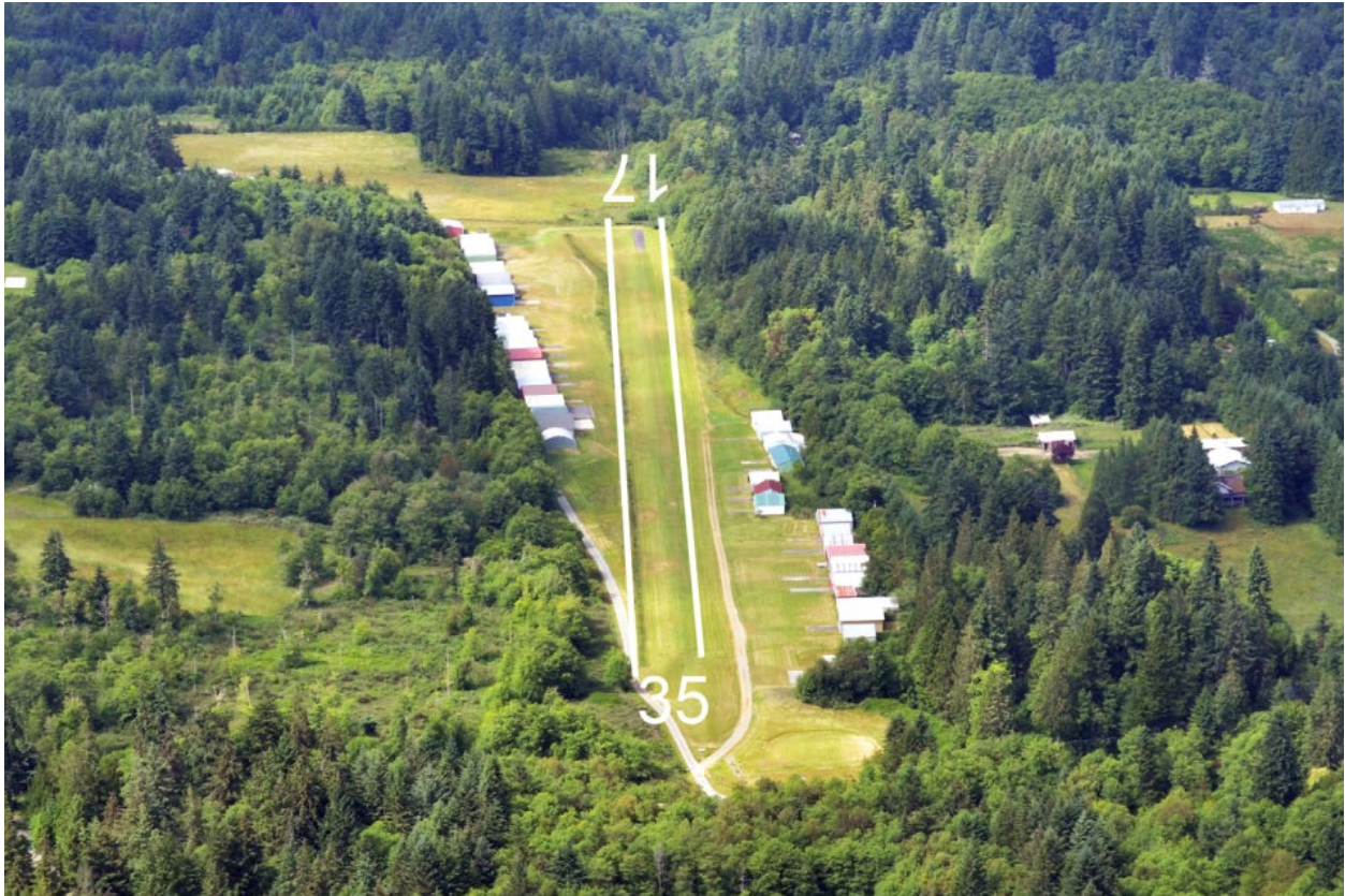
Figure 2-19. Vashon Municipal Airport
