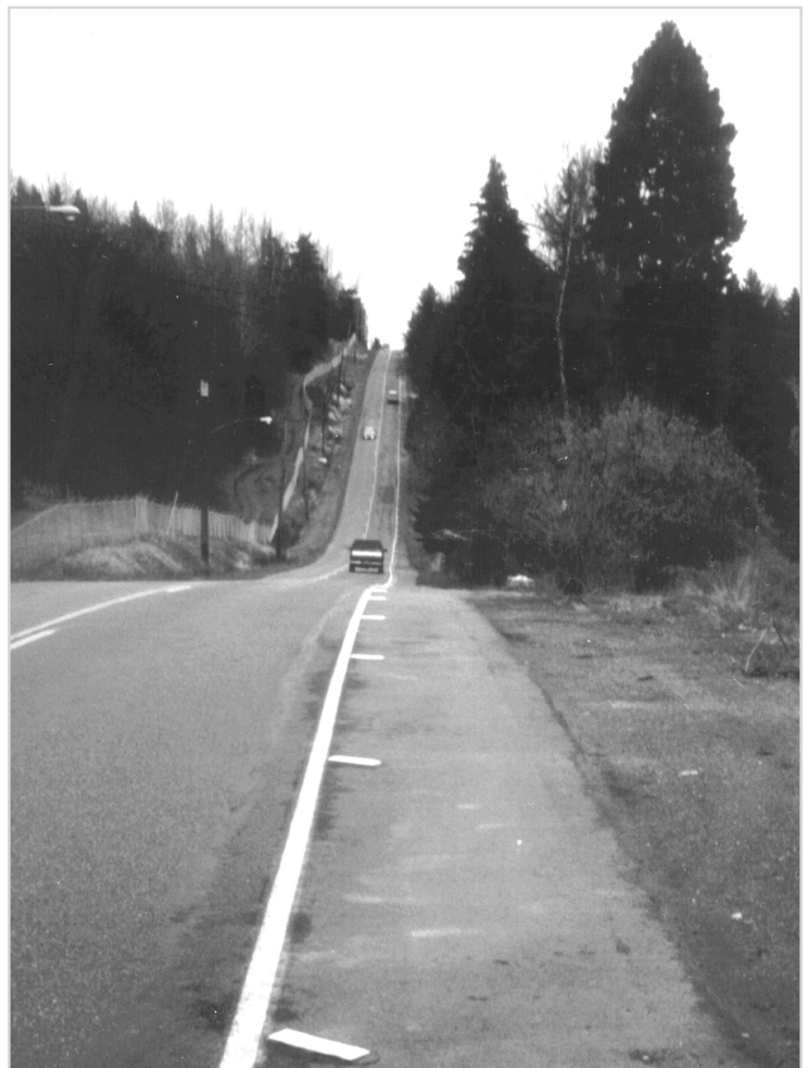
12th Ave. S. at the centerline of the proposed third runway on Feb. 24, 2000
