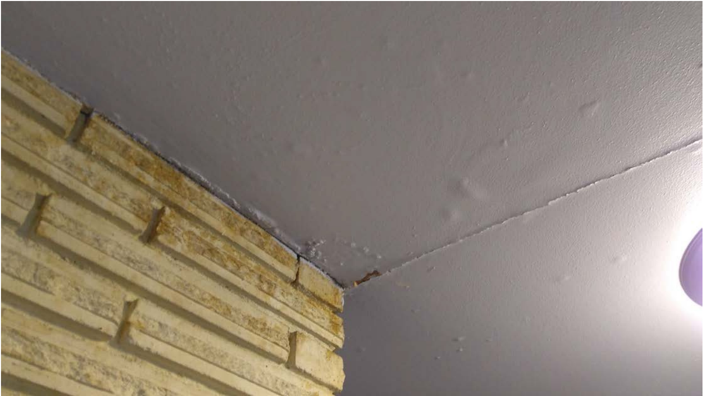
Black mold in attic Port Package-specific high density ceiling insulation. Many homes with this type of insulation develop moisture issues in the attic due to poor ventilation/HVAC design. This causes moisture which has migrated into the ceiling in the lower photo. At minimum, this requires replacement of both insulation and ceiling.
