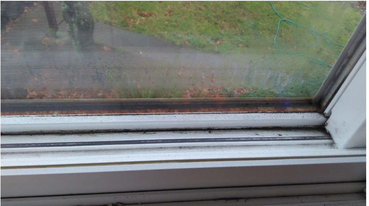
Corrosion. Once water finds a path between the panes, this becomes inevitable.
