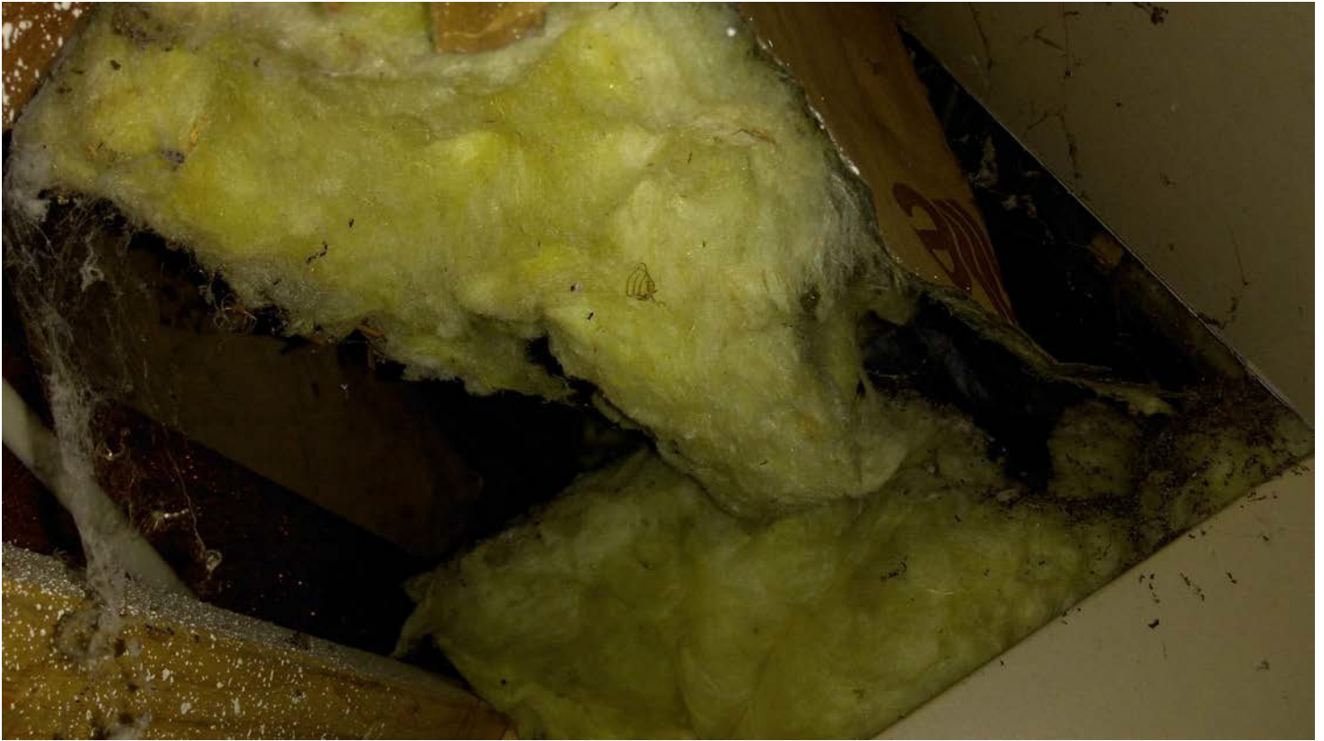
Black mold in attic Port Package-specific high density ceiling insulation. Many homes with this type of insulation develop moisture issues in the attic due to poor ventilation/HVAC design. This causes moisture which has migrated into the ceiling in the lower photo. At minimum, this requires replacement of both insulation and ceiling.
