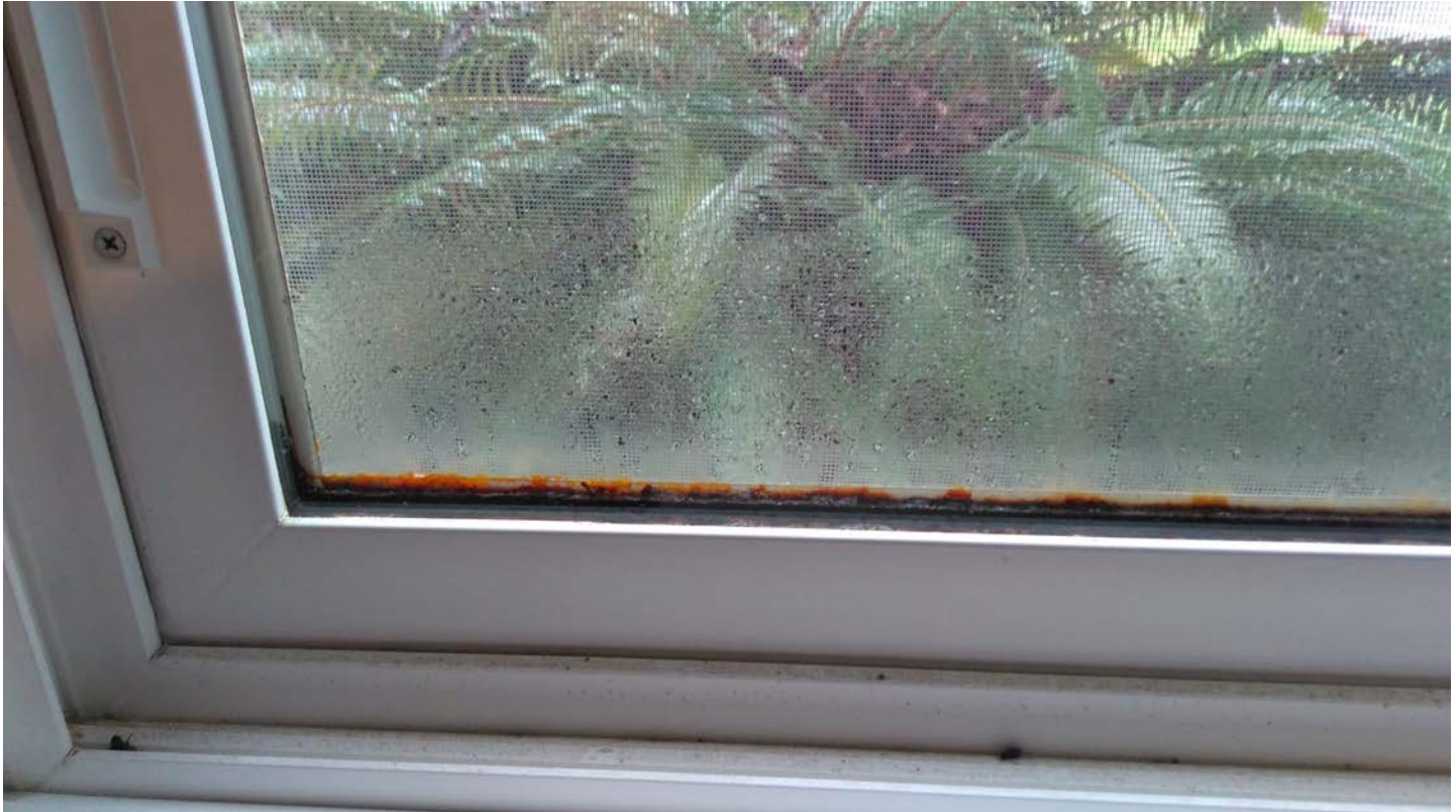
Corrosion. Once water finds a path between the panes, this becomes inevitable.
