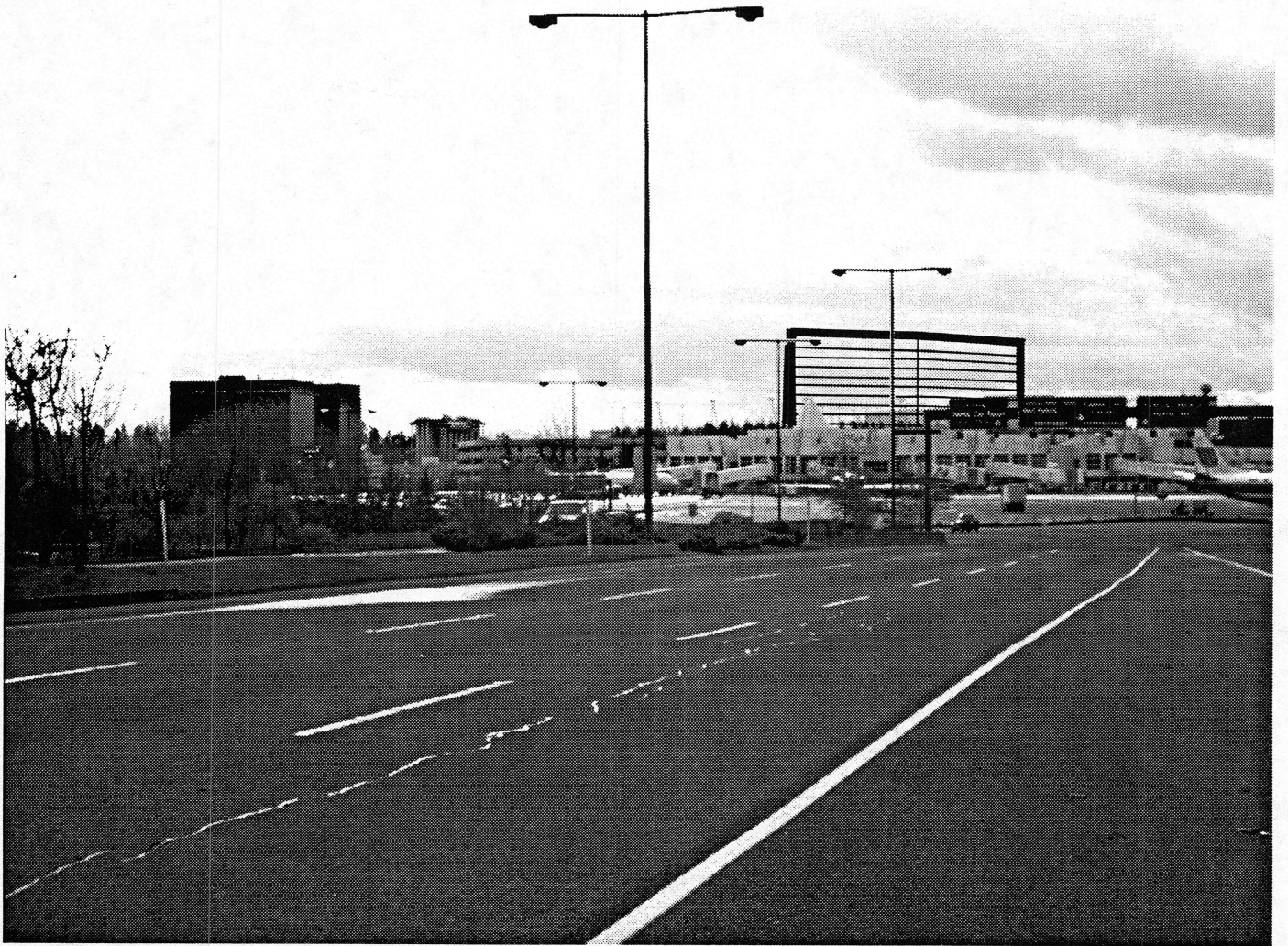
North Access Road
