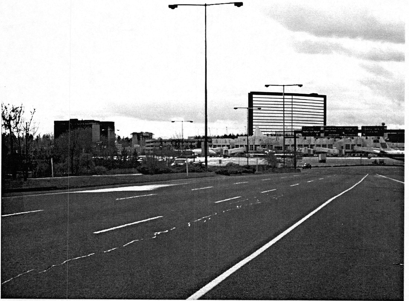
North Access Road
