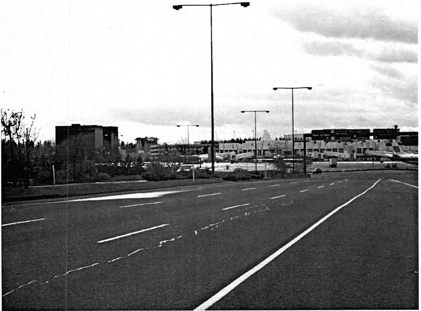
North Access Road
