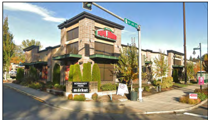
Figure 2.14 Normandy Park Towne Center Entrance (photo courtesy of Google Earth)
