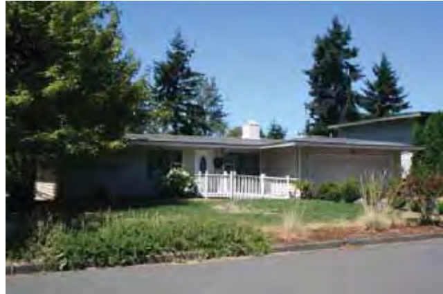
East (front) and south elevations
