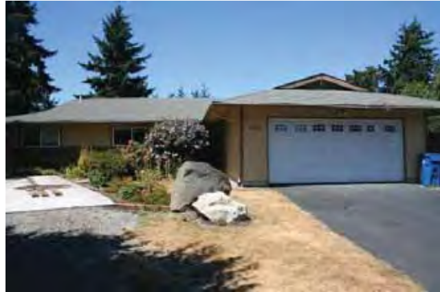
East (front) and south elevations
