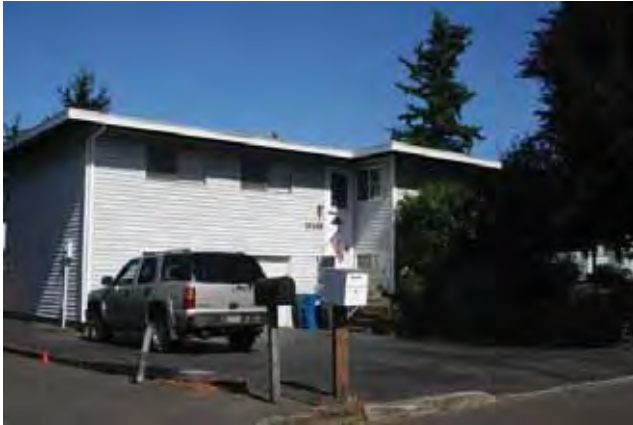
East (front) and south elevations
