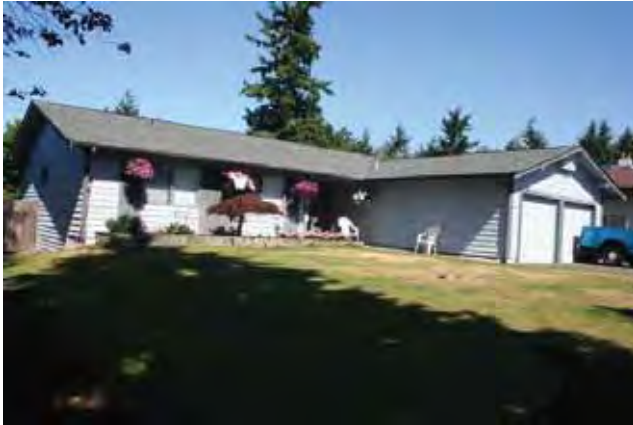
East (Front) and south elevations
