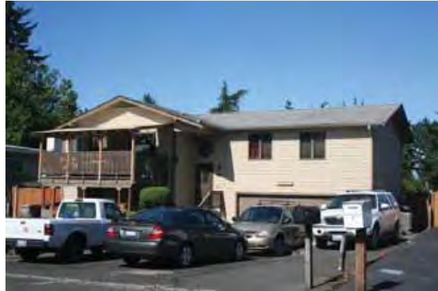
East (front) and north elevations
