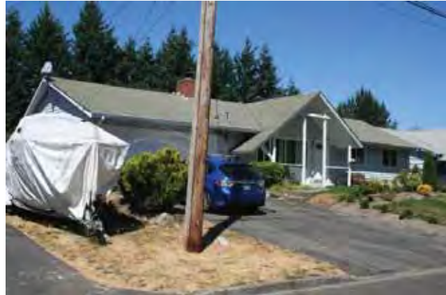
East (front) and south elevations
