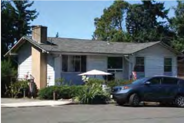
Southeast (front) and southwest elevations
