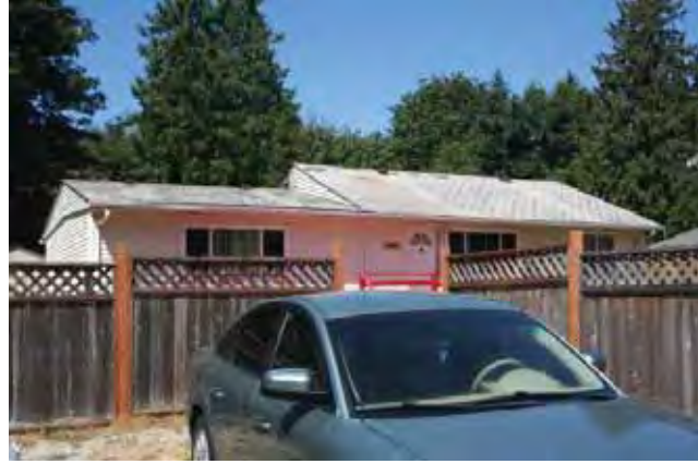
South (front) and west elevations
