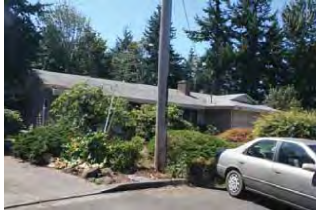
East (front) and south elevations
