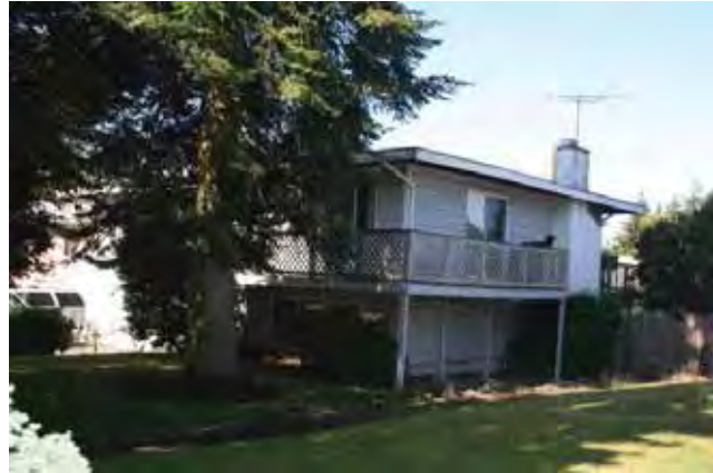
East (front) and north elevations
