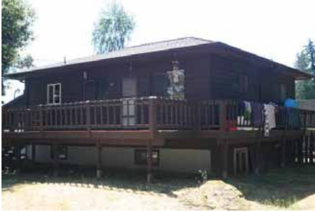
East (front) and north elevations
