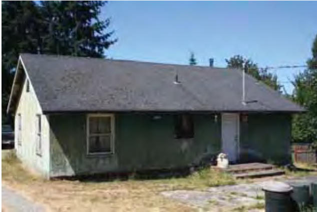
East (front) and south elevations
