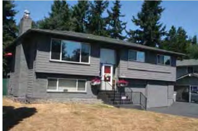
East (front) and south elevations
