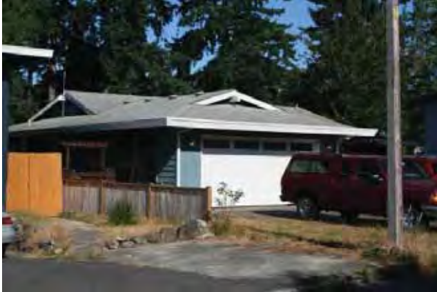
East (front) and south elevations
