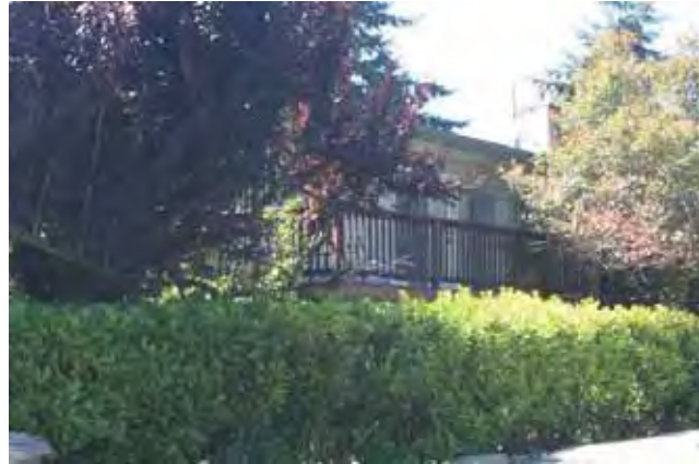
East (front) and north elevations
