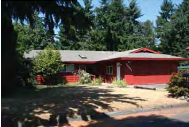
East (front) and south elevations
