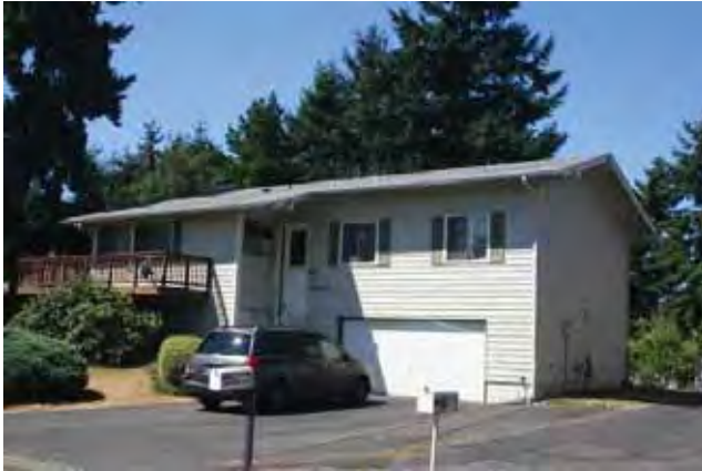
East (front) and north elevations
