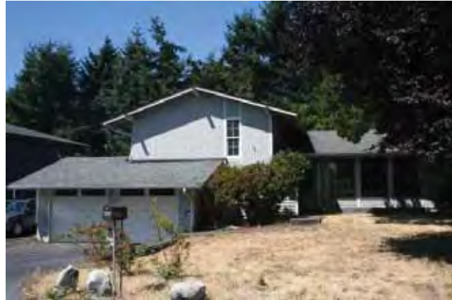
East (front) and north elevations
