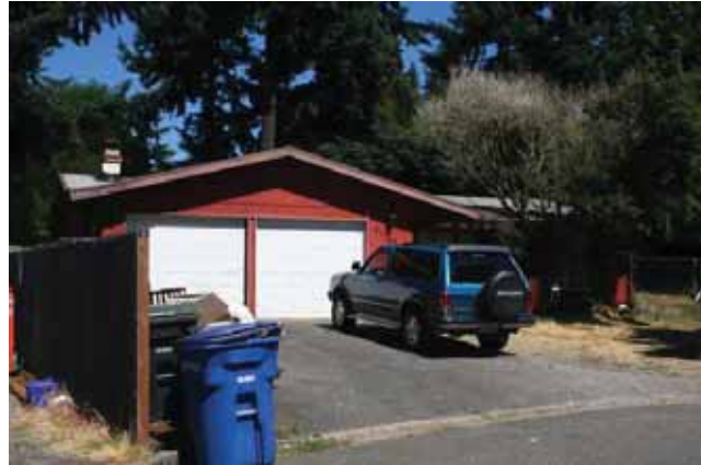
East (Front) and south elevations
