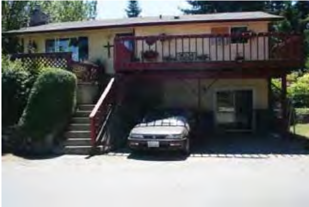
North (front) elevations
