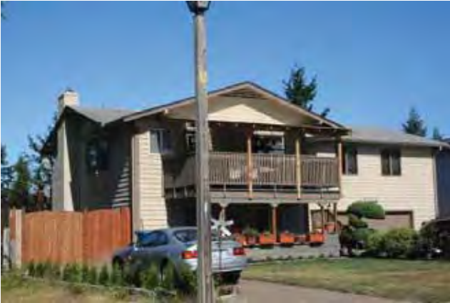
East (front) and south elevation
