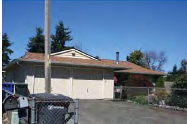
East (front) and south elevations
