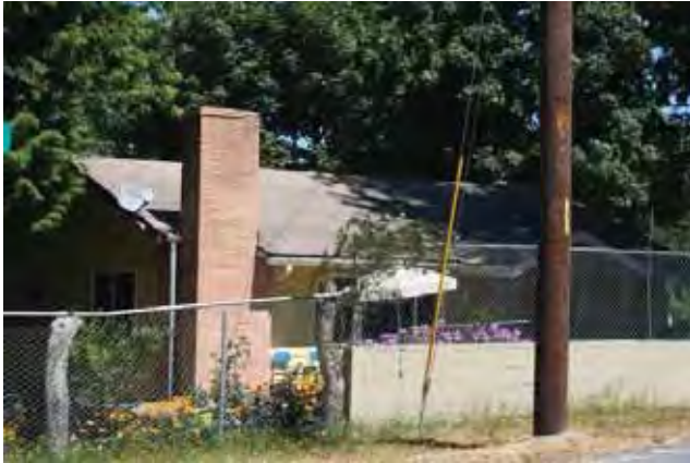
South (front) and west elevations
