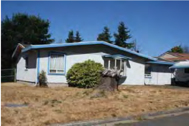
East (front) and south elevations
