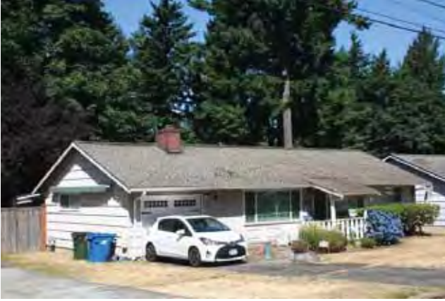
East (front) and south elevations
