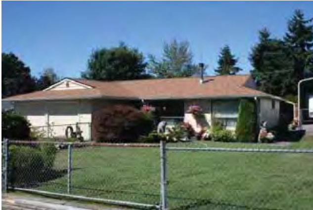
East (front) and north elevations
