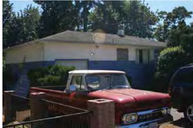
North (front) and east elevations
