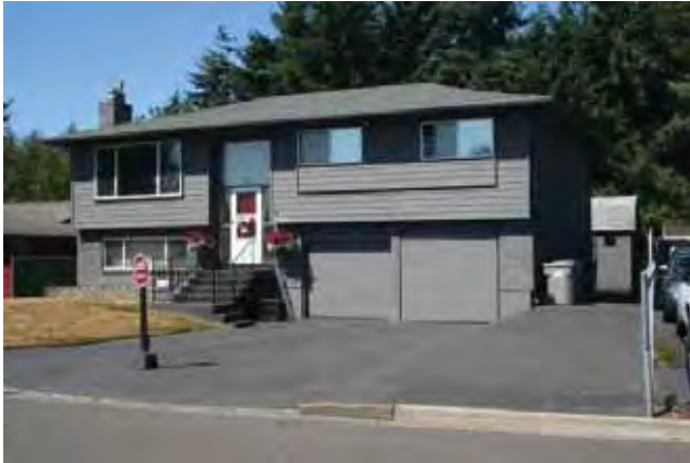
East (front) and north elevations
