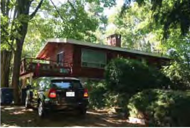
East (front) and south elevations
