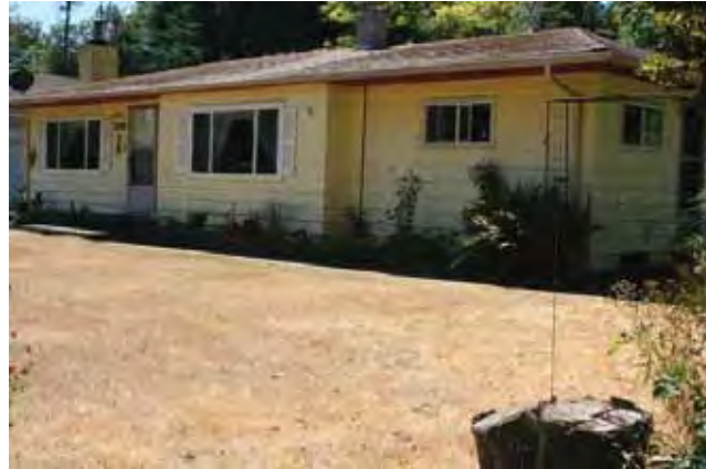
East (front) and north elevations
