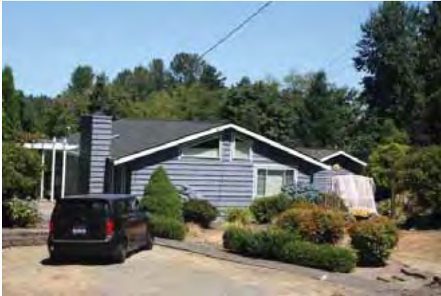
South and west (front) elevations
