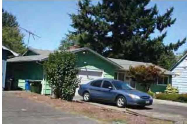
East (front) and south elevations
