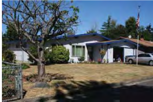
East (front) and south elevations
