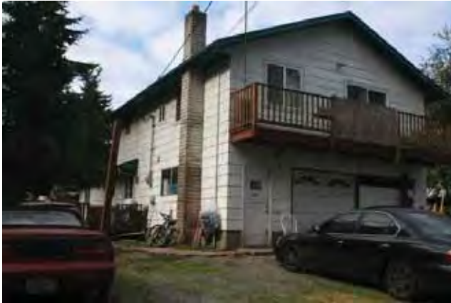
North (front) and east elevations
