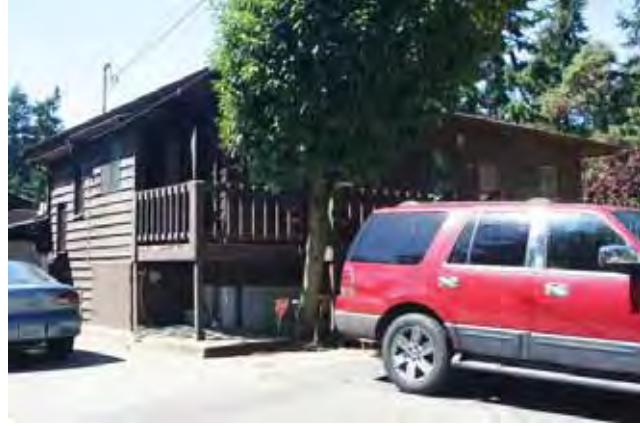
East (front) and south elevations
