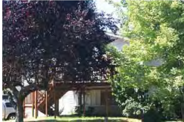
East (front) and north elevations
