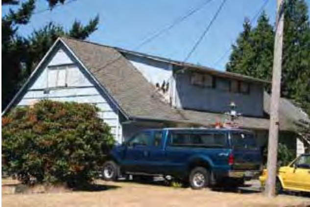
East (front) and south elevations
