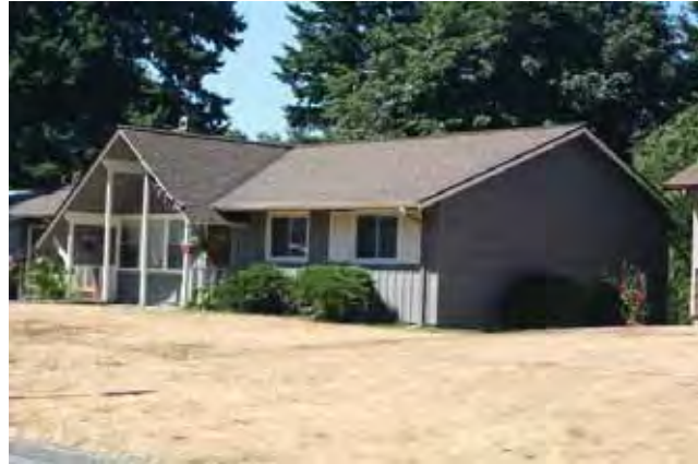
East (front) and north elevations
