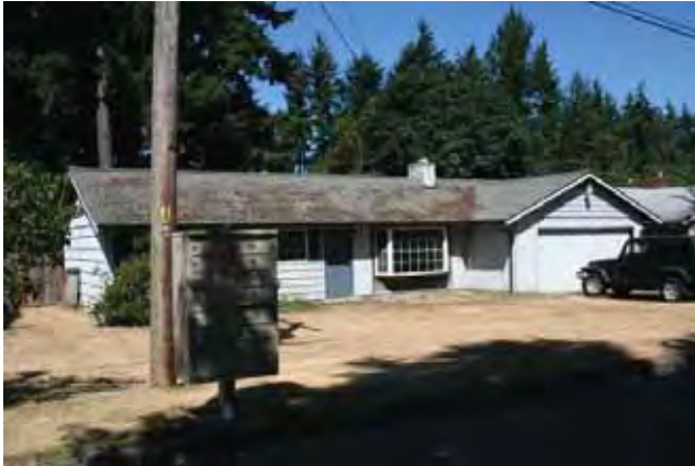
East (front) and south elevations
