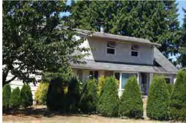
East (front) and south elevations
