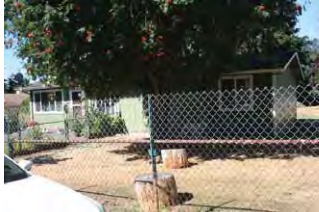
East (front) and north elevations
