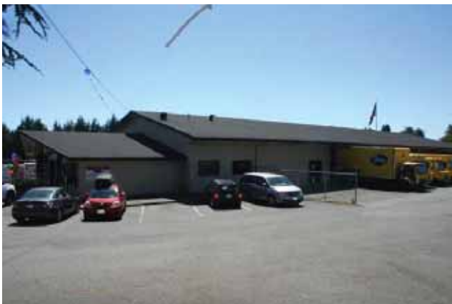
East (front) and north elevations
