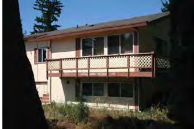
East (front) and north elevations
