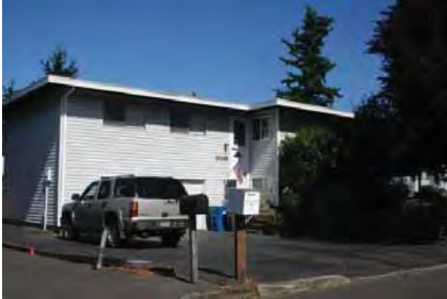
East (front) and south elevations
