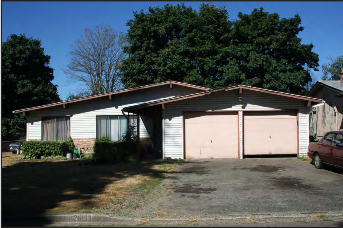
Figure 17. The Mountha House at 21853 32nd Place South, east elevation, view to the west.
