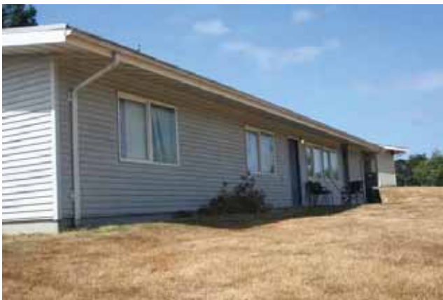
North (rear) and east elevations
