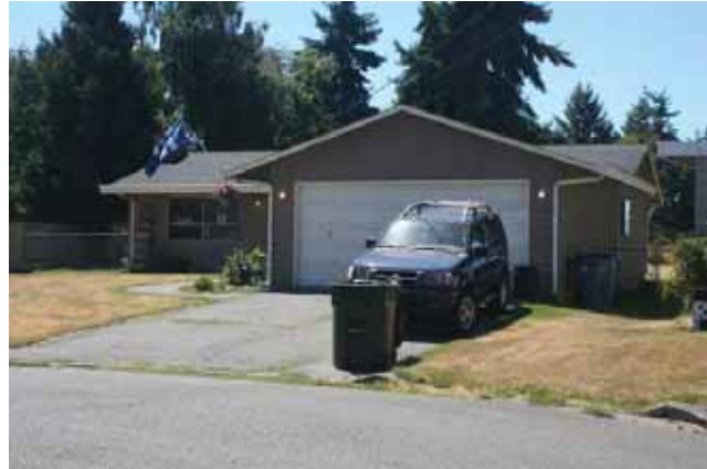
Northeast (front) and northwest elevations
