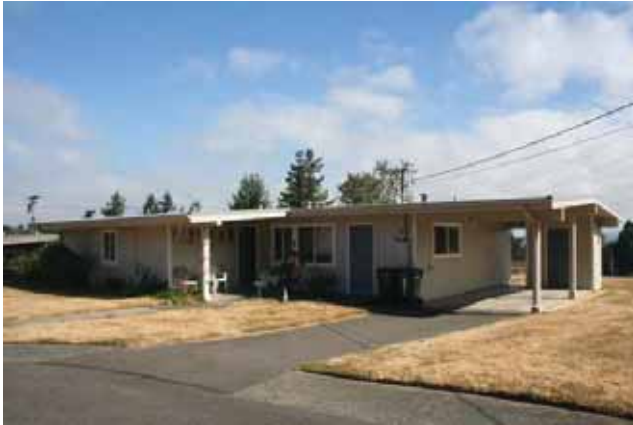
Southwest (front) and southeast elevations
