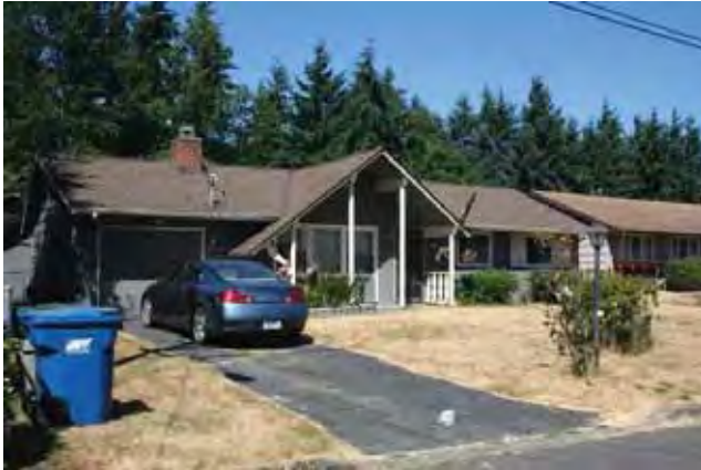
East (front) and south elevations
