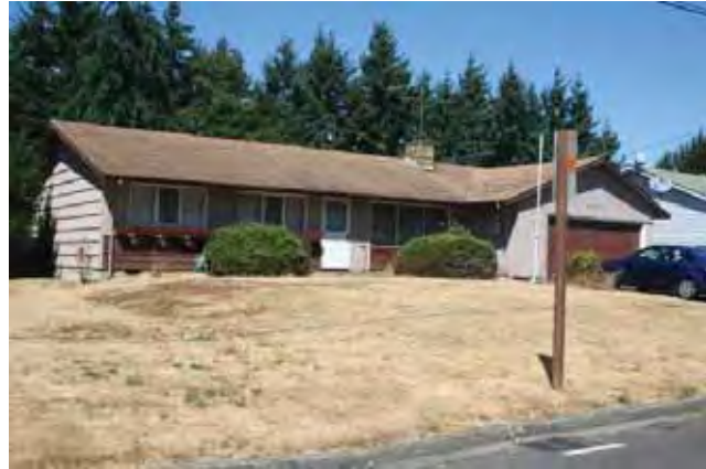
East (front) and south elevations
