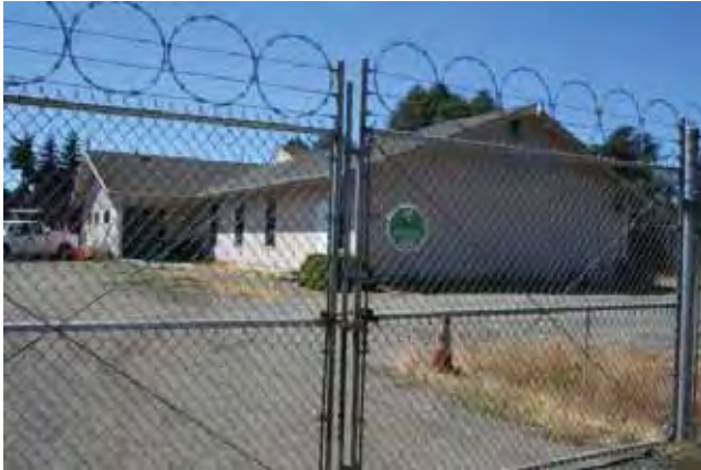
South and east elevations
