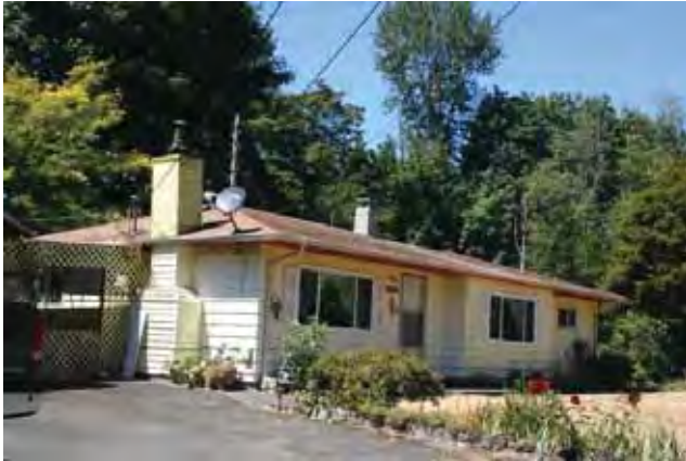
East (front) and south elevations
