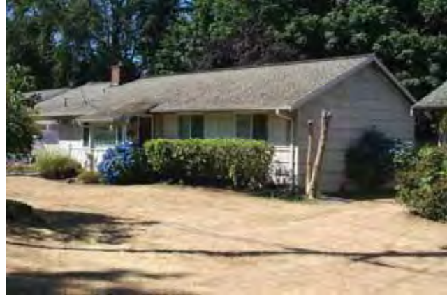
East (front) and north elevations
