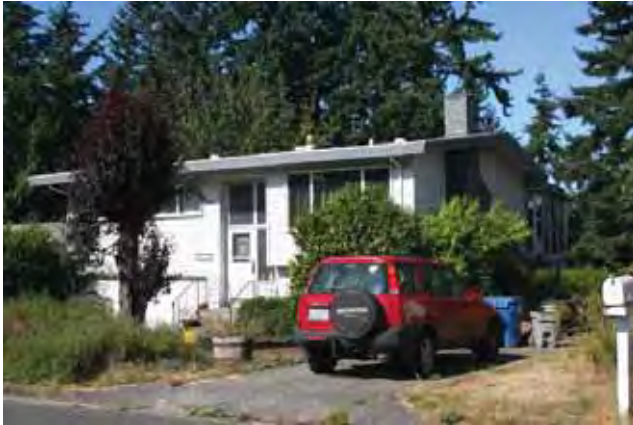
East (front) and north elevations
