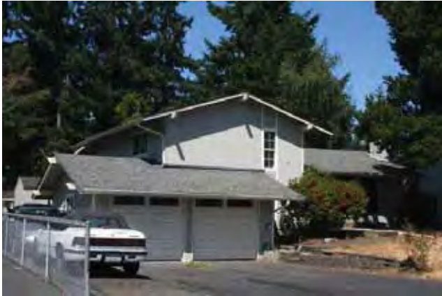
East (front) and south elevations
