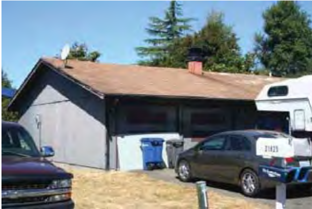
East (front) and south elevations
