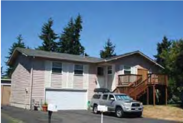
East (front) and south elevations
