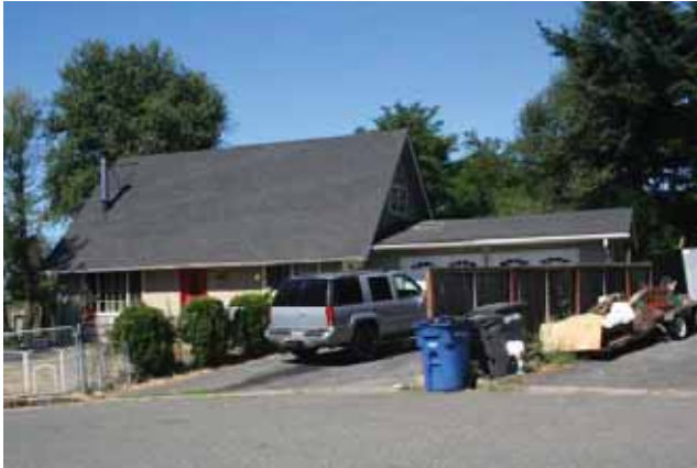
East (front) and north elevations
