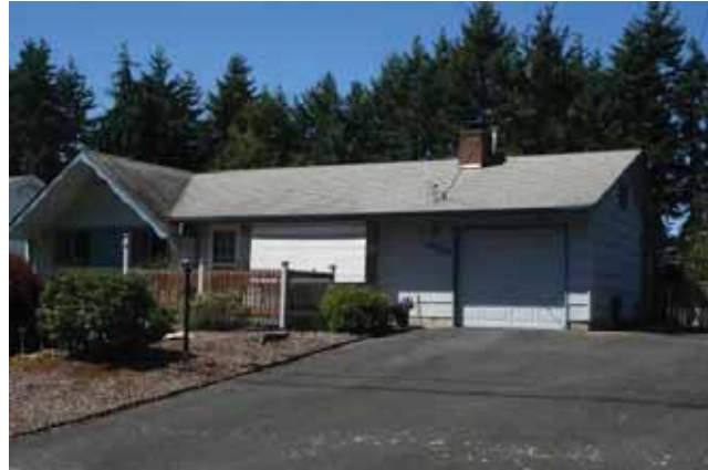
East (front) and north elevations
