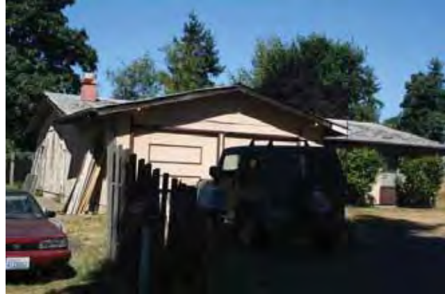
East (front) and south elevations
