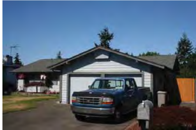
East (front) and north elevations
