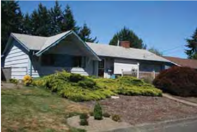
East (front) and south elevations
