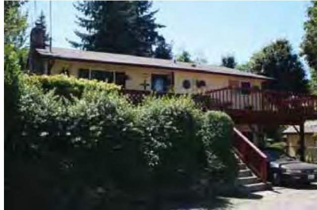
North (front) and east elevations
