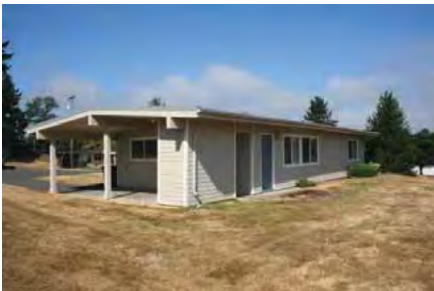
Northeast (rear) and northwest elevations
