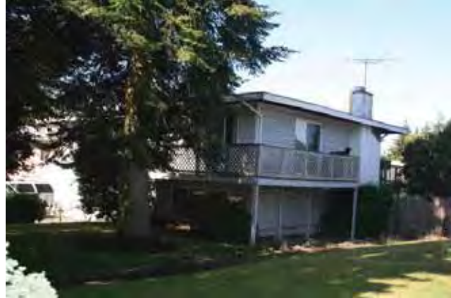
East (front) and north elevations
