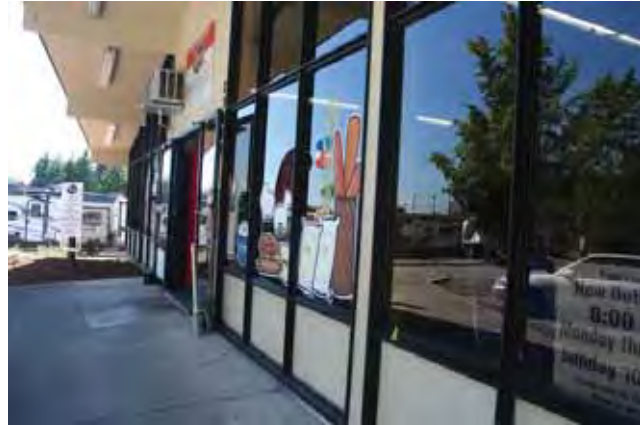
East (front) elevation, storefront detail
