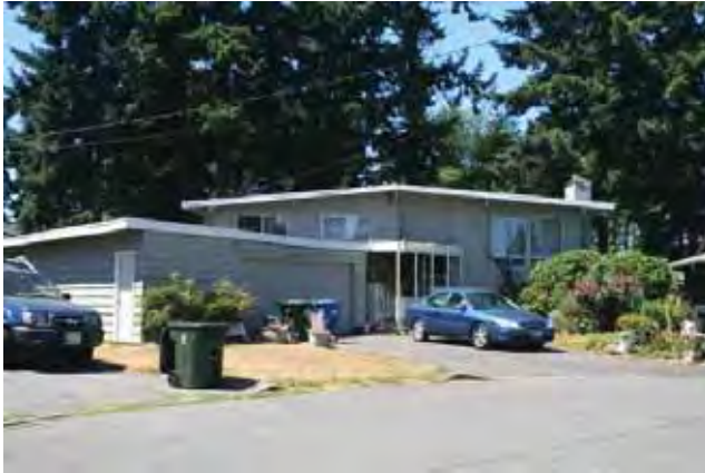
East (front) and south elevations
