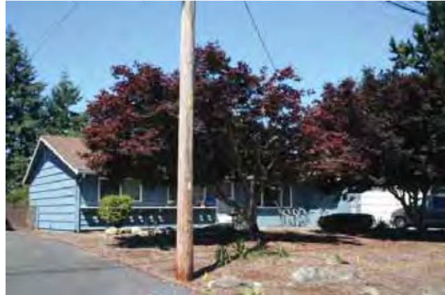
East (front) and south elevations
