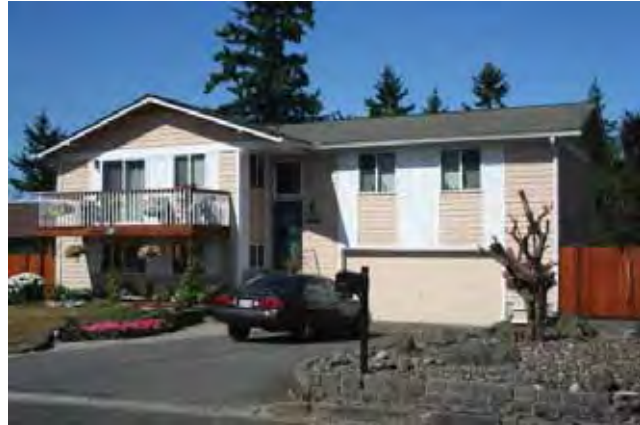
East (front) and north elevations
