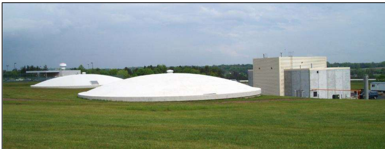
Figure 8: Buried AWWA D110 Type III Tank at Akron-Canton Airport
