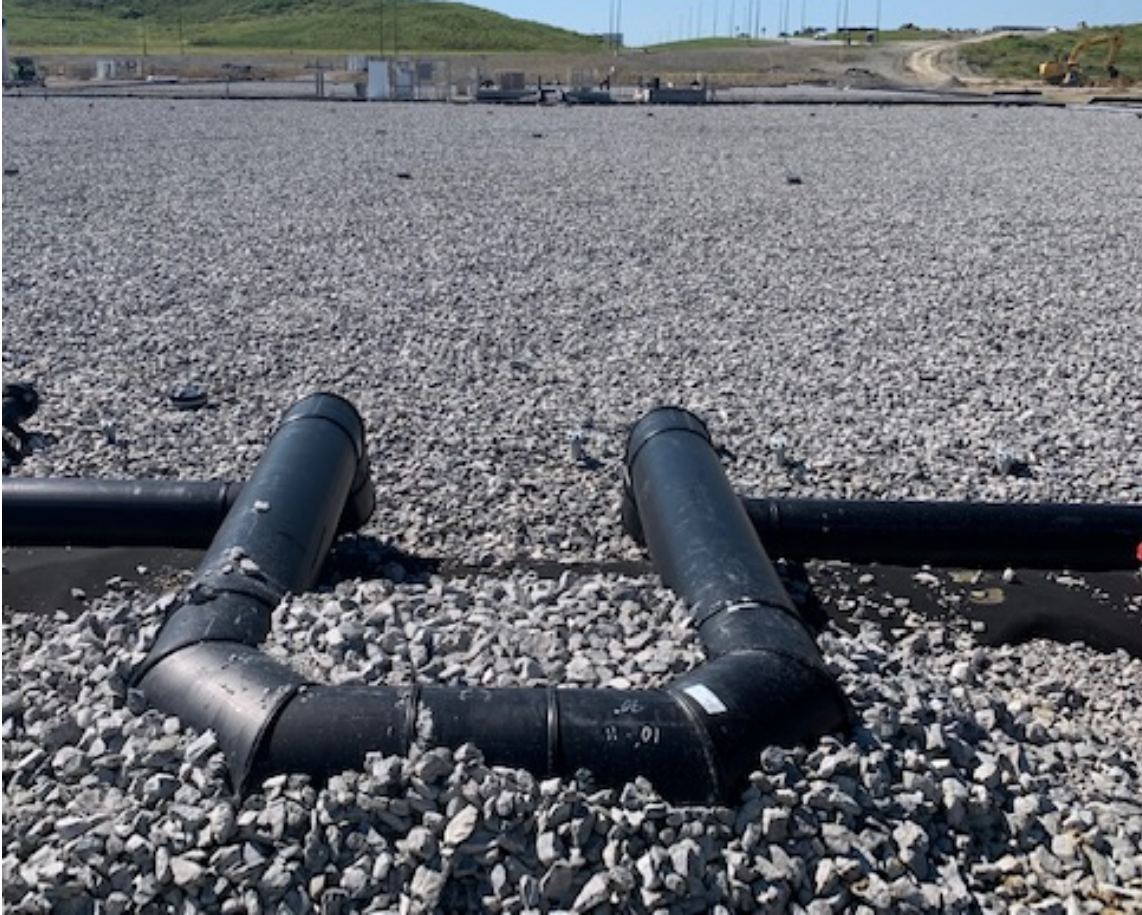
Figure 2. Aerated Gravel Bed Cell.
