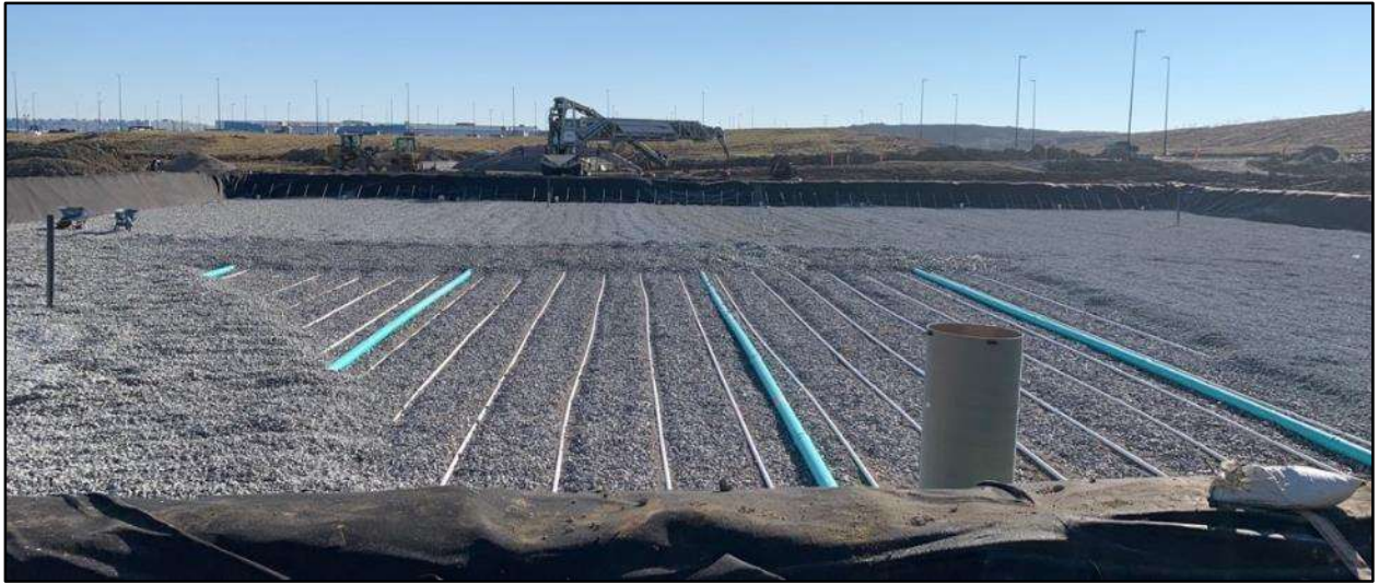
Figure 15: Drain Lines and Air Diffusers During Construction
