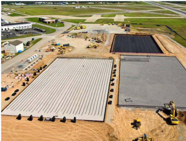
Figure 2. Construction of the BNIA Aerated Gravel Bed.
