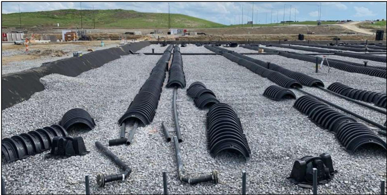
Figure 14: Influent Dosing Lines and Infiltration Chambers During Construction
