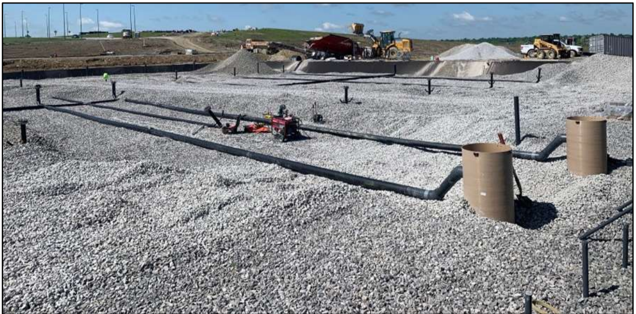
Figure 16: Recirculation Lines and Sumps During Construction
