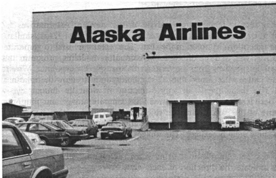
J. Existing Alaska Hangar and Shop
