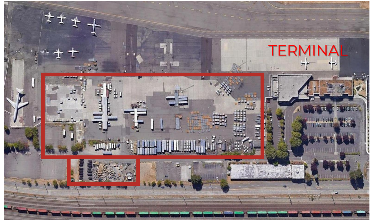
KCIA Air Cargo Facilities and Pass. Terminal
