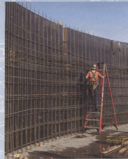
Above, a worker assembles a curving helix wall for SeaTac's consolidated rental car facility. Below, an artist's rendering shows what the completed structure will look like when it opens two years from now.
