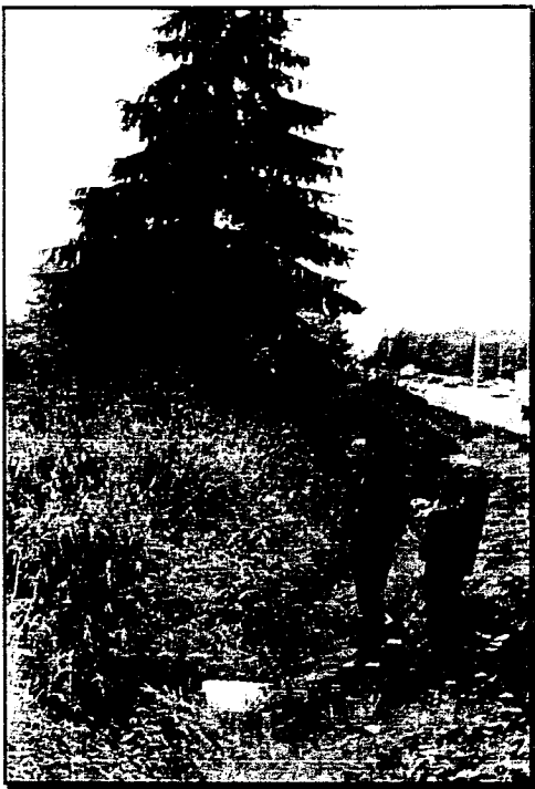
NEPL on SR 518 (landmark is fir tree, 24" CMP) 1
