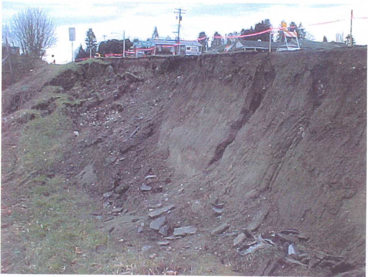
View to east showing slide along the northern edge of the Martin Way earth embankment slide. The maximum vertical offset of the headscarp at this area was 3.3 m (GPS N47.04693 W122.85092; 1000 03/04/01).
