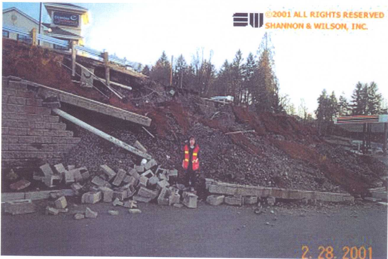
Note broken water pipe at the top of slope (GPS N47.02479 W122.92230; 02/28/01).
