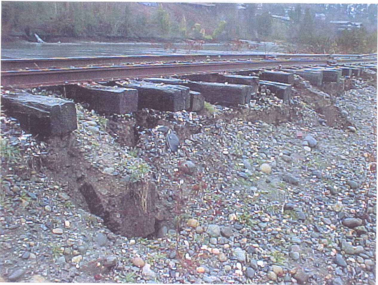
Slumping of railroad embankment in Olympia. Tracks are supported by a wooden trestle that underlies the embankment (GPS N47.04567 W122.91043; 1230 03/01/01).
