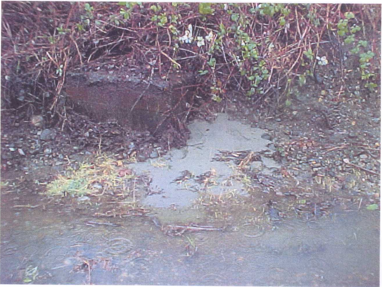
Sediment ejecta at base of embankment shown previously indicating liquefaction (GPS N47.0402 W122.8939; 1630 03/01/01)
