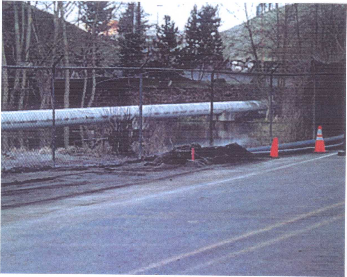
Figure 11. Sewer main repair at south abutment (GPS N47.1917° W122.5733°; 0737 03/04/01)
