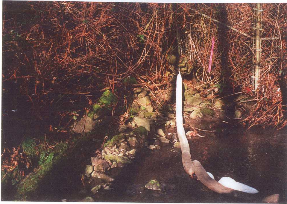
Figure 1. Absorbent boom in stream below SDS1 outfall. Photo taken by P. Willing, January 28, 2002.
