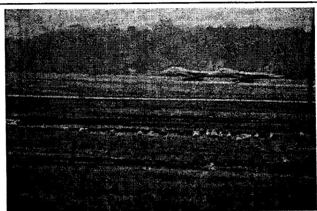
All areas of standing water on the airport operating area should be drained to discourage bird use. (Photo courtesy USAF)
