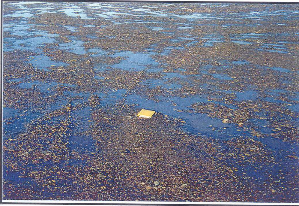
Exhibit I: Standing water on the top of the fill embankment at about South 160 th Street, 28 January 2002
