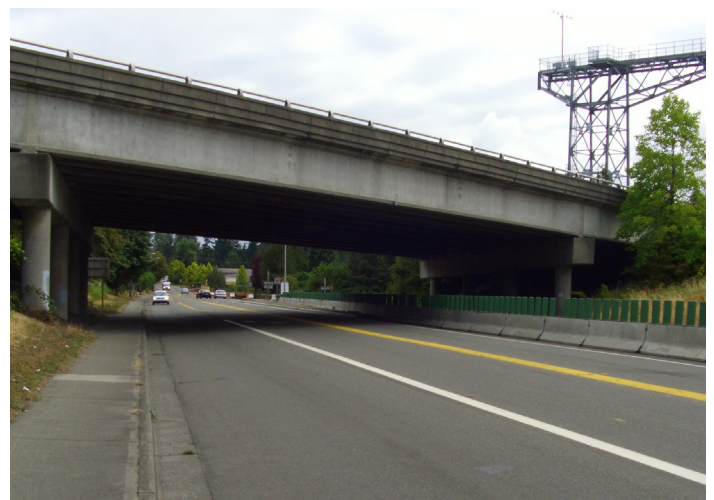
Des Moines Memorial Drive South at SR 518
