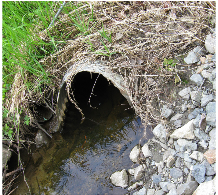
Existing stormwater infrastructure in the NERA
