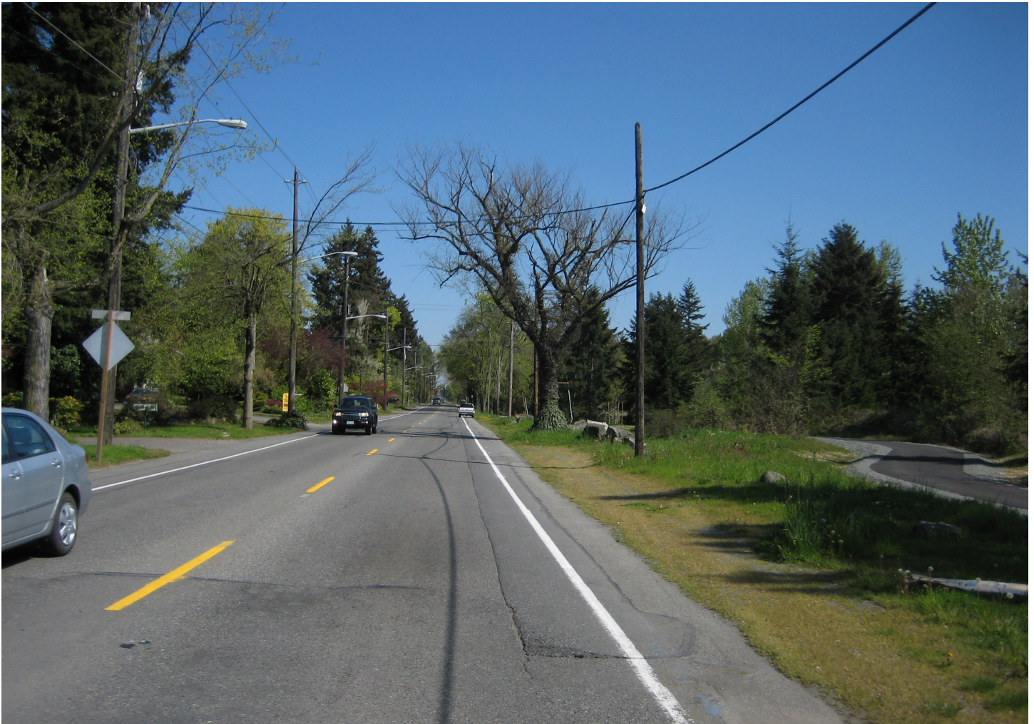
Des Moines Memorial Drive with adjacent SeaTac Sunset Park Trail
