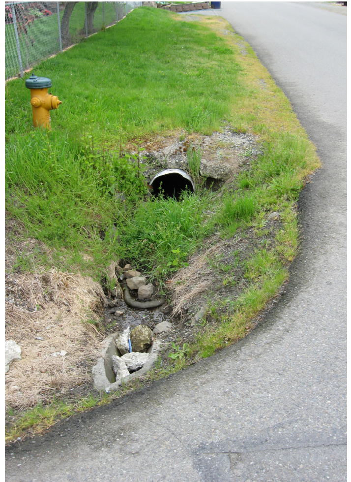
Roadside ditch drainage
