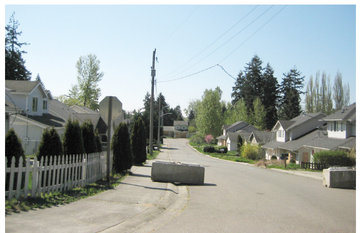
Abandoned Port-owned single-family homes in Subarea 4 that have since been demolished
