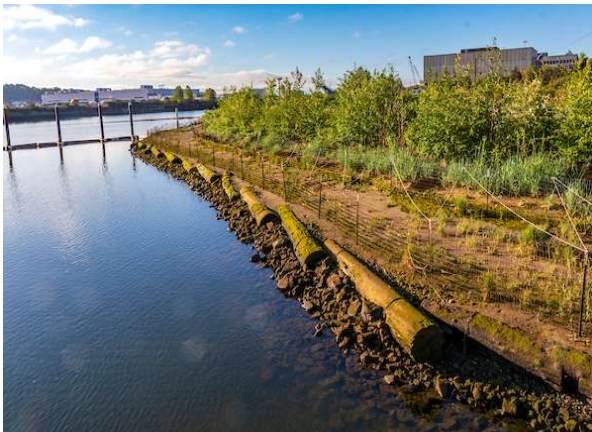
Green Shoreline Stabilization
