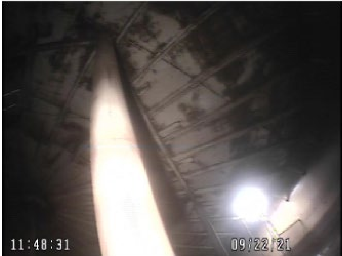
Significant rust on interior tank surfaces
