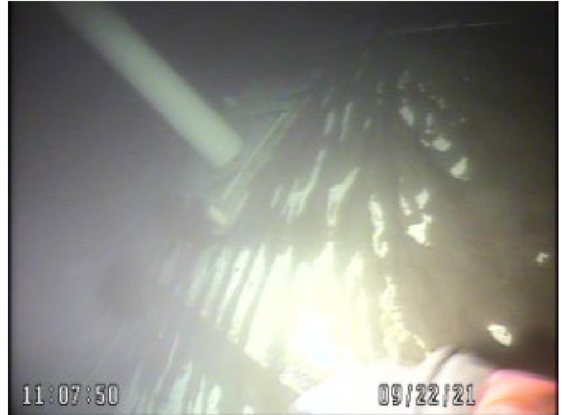
Significant rust on interior tank surfaces
