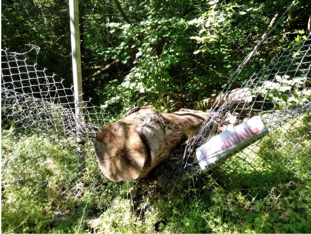
Photo 13: Miller Creek Buffer – Fence line maintenance noted, large tree laying on fence.
