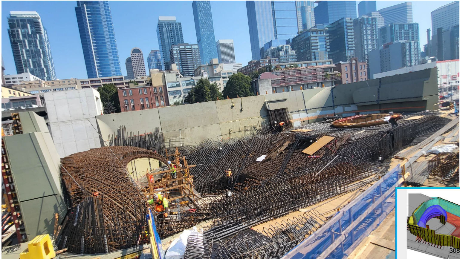
The Reef forming and rebar installation
