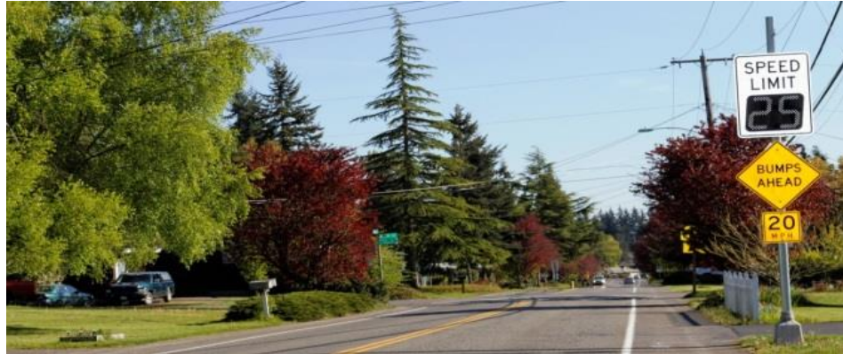
Figure T-4: 8th Avenue S south of S 312th Street
