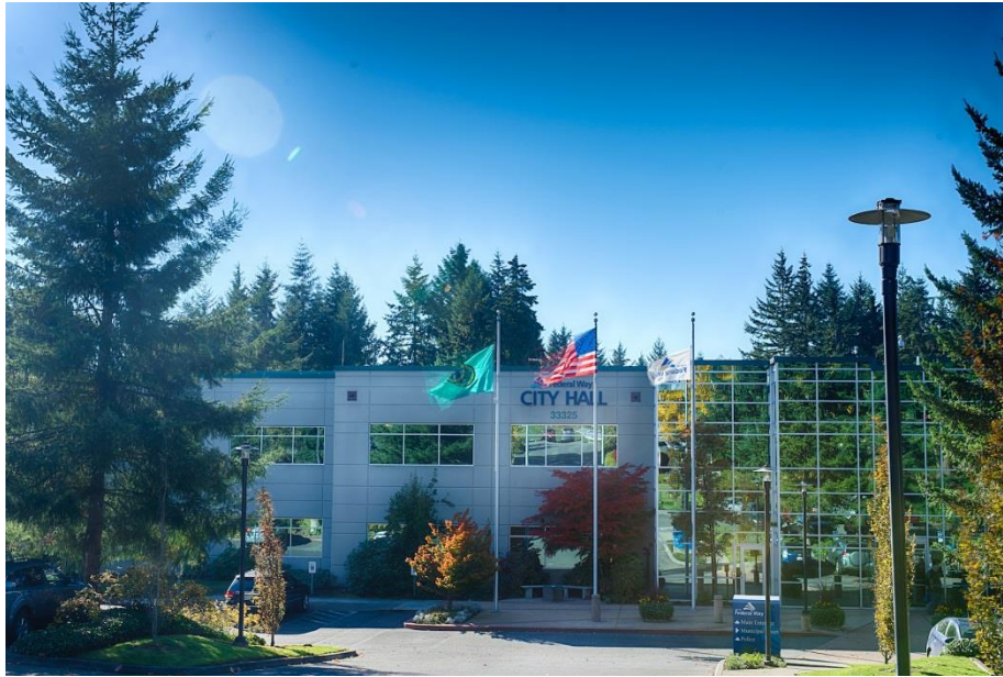
Source: City of Federal Way
