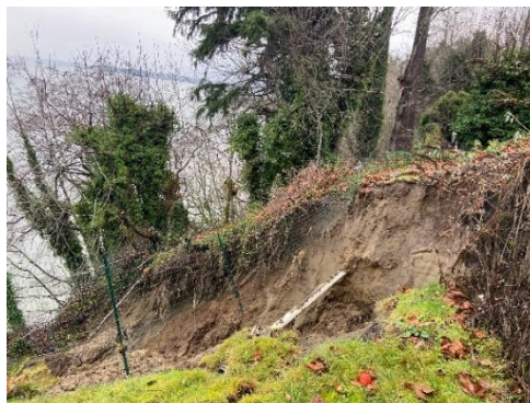
Figure CCR-9: Landslide along the Federal Way shoreline
