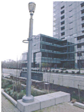
Pedestrian area lighting
