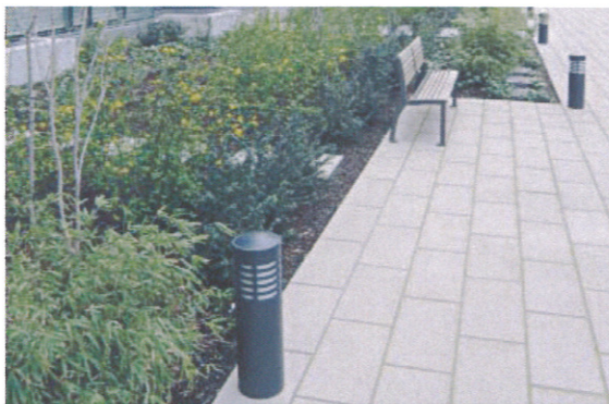
Use of bollards as pedestrian pathway lighting
