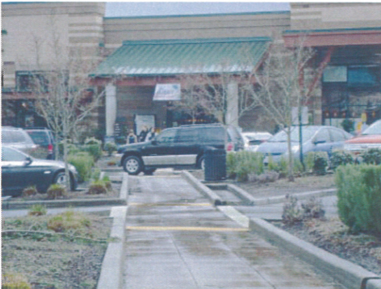
Pedestrian paths integrated with landscaping provide a safe path for pedestrians.
