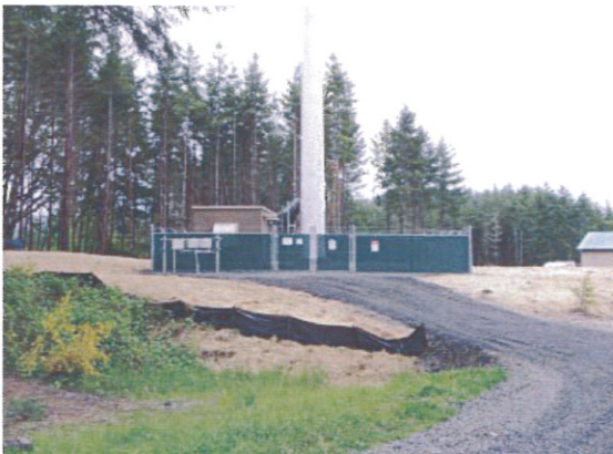
Ground mounted facilities shall provide a shelter and screened enclosure to minimize visual impact.
