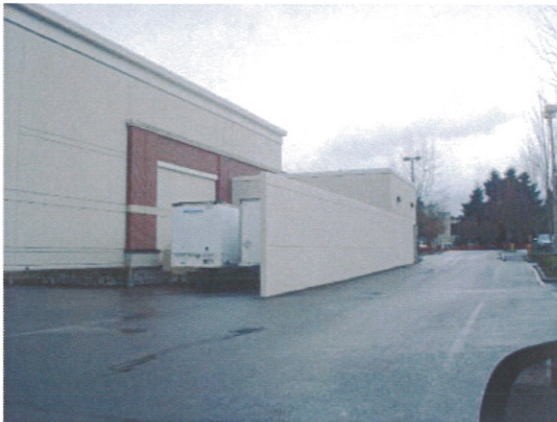
Use of wall matching the character of building to screen loading area.
