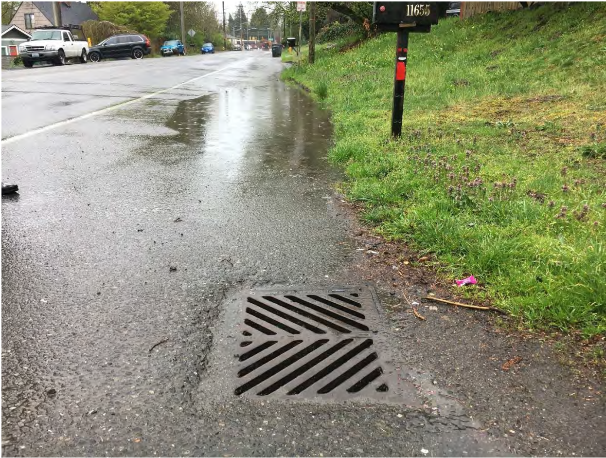
FIGURE 1: Looking southeast, picture taken 4/5/2019, west side of Glendale Way S, CB10460, flow direction towards southeast
