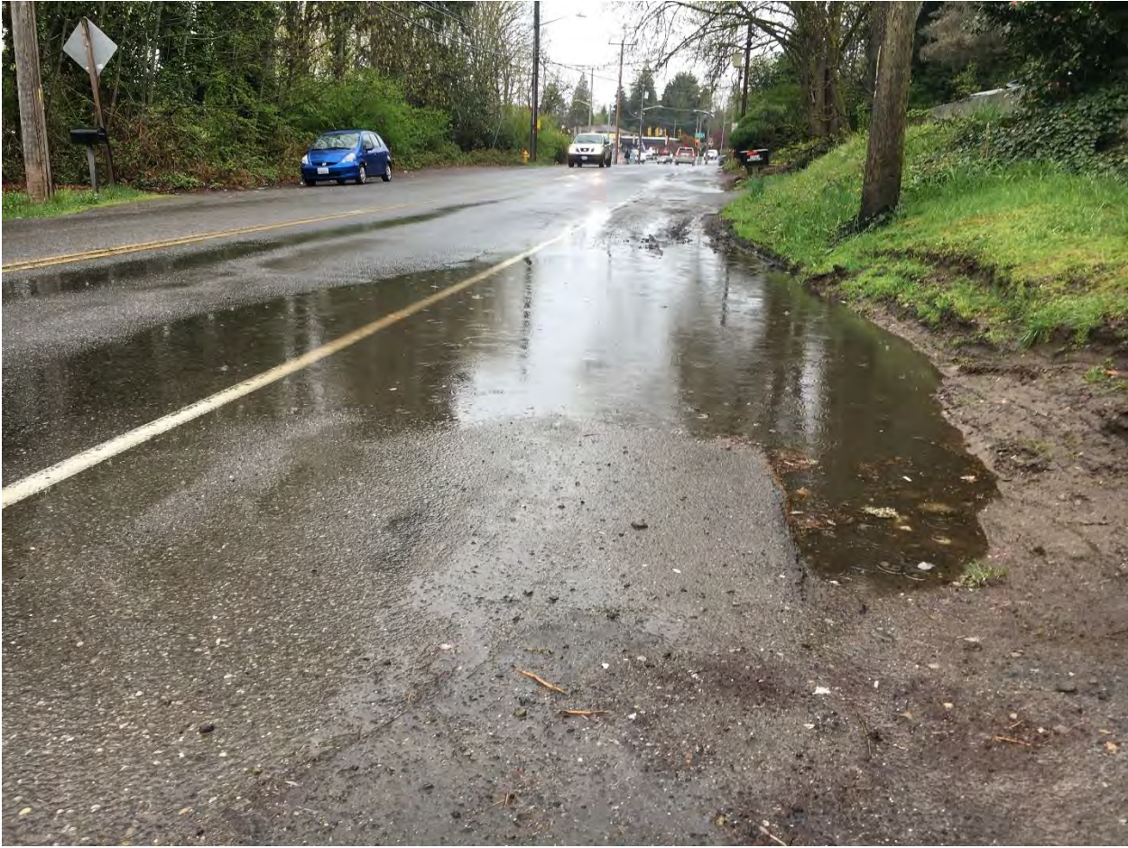
FIGURE 2: Looking southeast, picture taken 4/5/2019, west side of Glendale Way S, flow direction towards southeast
