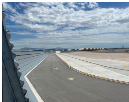
44 Tucson Int'l Leverages Partnerships and Federal Funding to Enhance Airfield Safety
