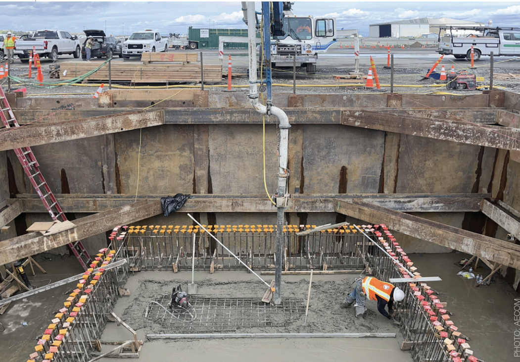
Crews pour the bottom slab for the new fuel vault, which is buried 15 feet deep.
