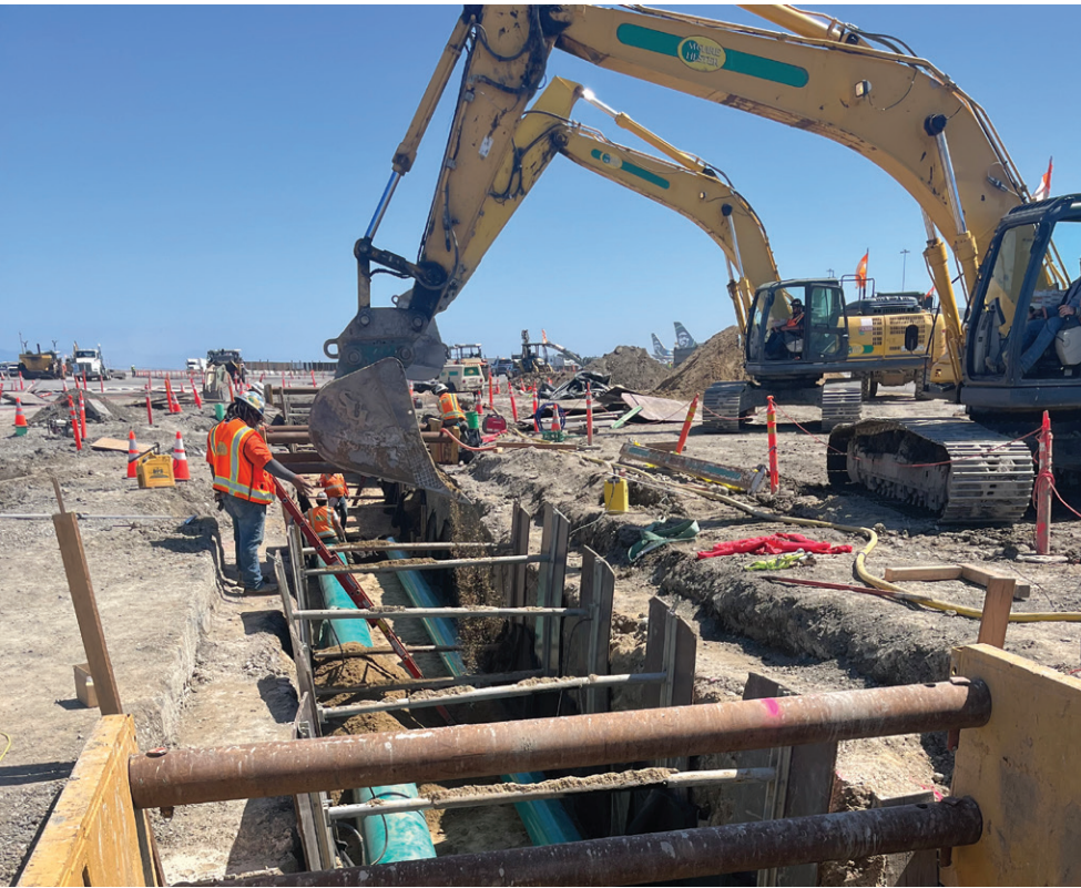
8 Taxiway Reconstruction Project Improves Safety at San Francisco Int'l
