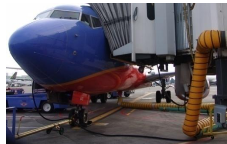
Pre-conditioned air and 400Hz being supplied at gates
