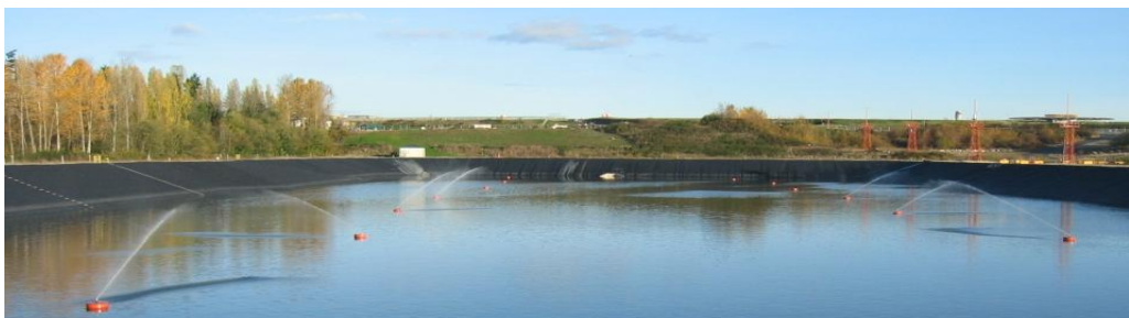
Sea-Tac Airport stormwater pond
