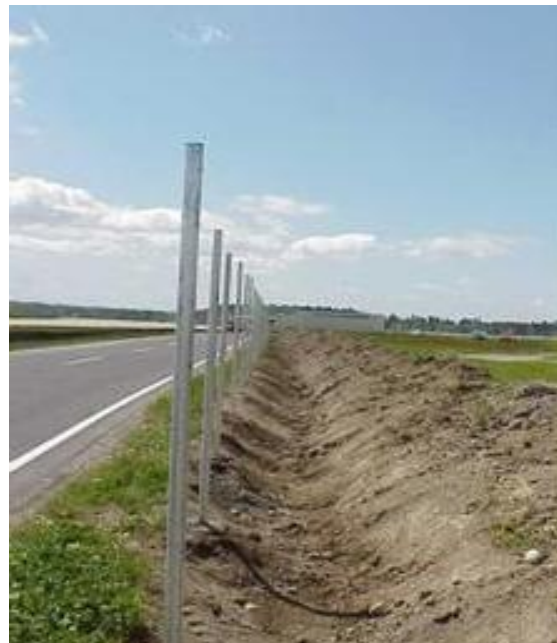
Installation of coyote deterrent fence
