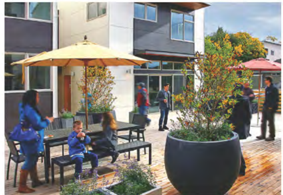
Marion Green Townhomes – Townhomes built around a shared courtyard space with parking underneath – providing single-family housing at three times the density.
