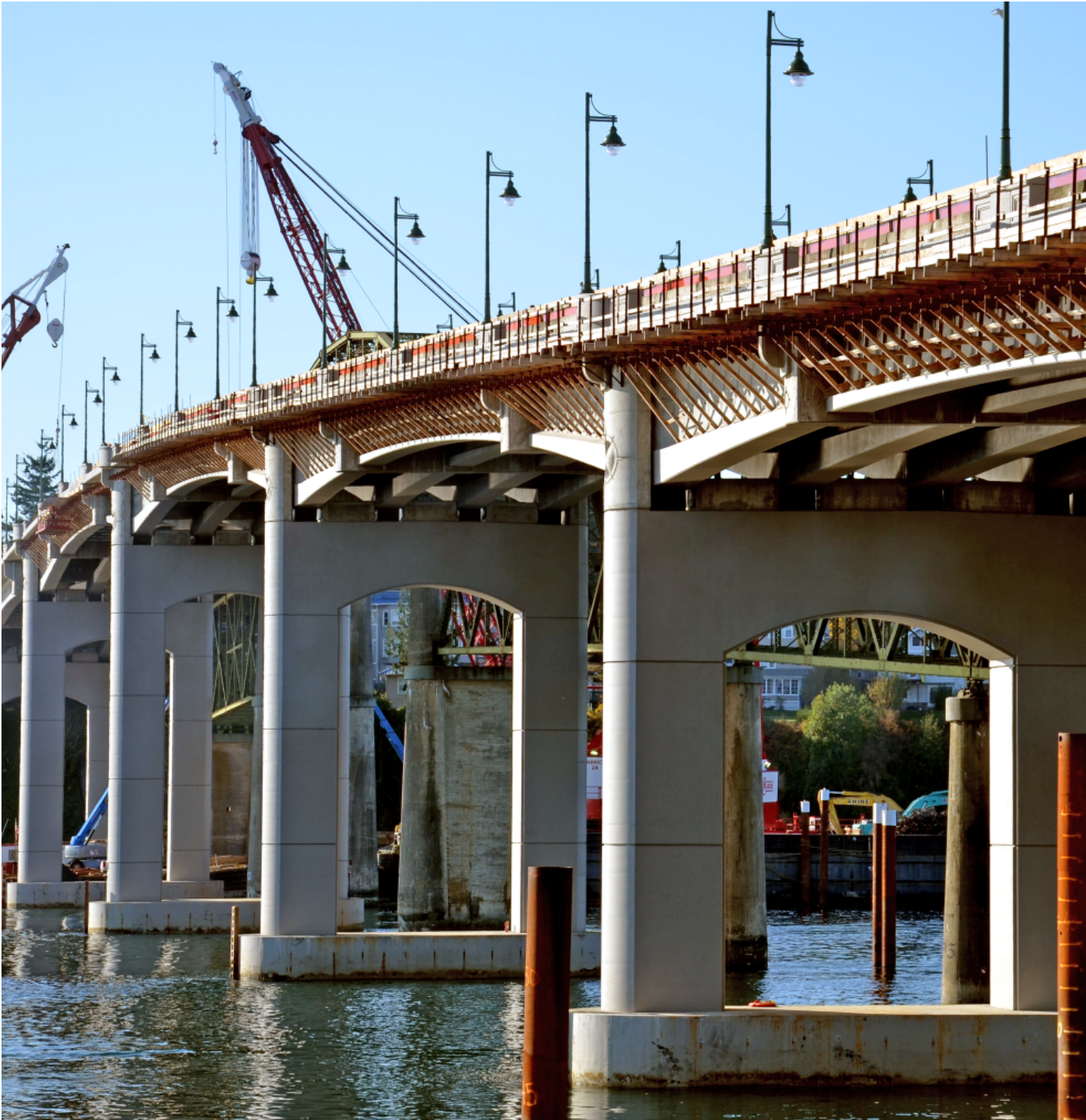
The new Mannette Bridge in Bremerton opened November 10, 2011.
