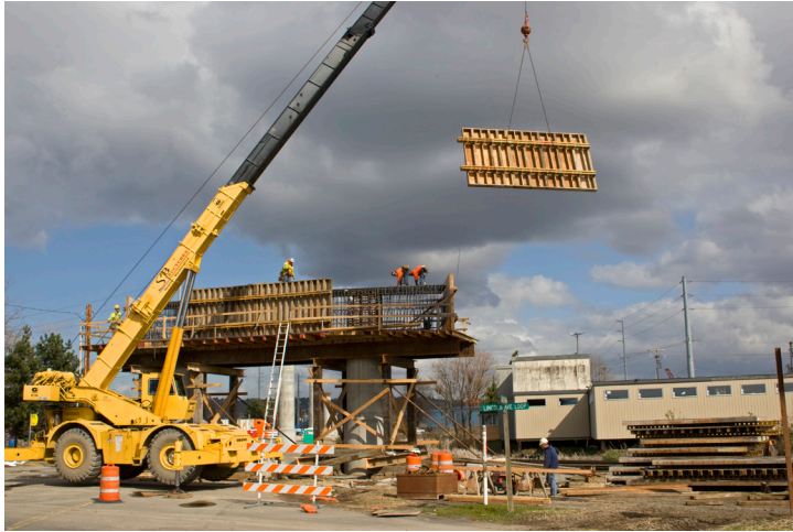
City of Tacoma, Lincoln Avenue Overpass
