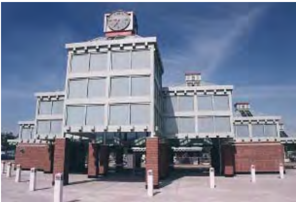
City of Auburn Commuter Rail Station
