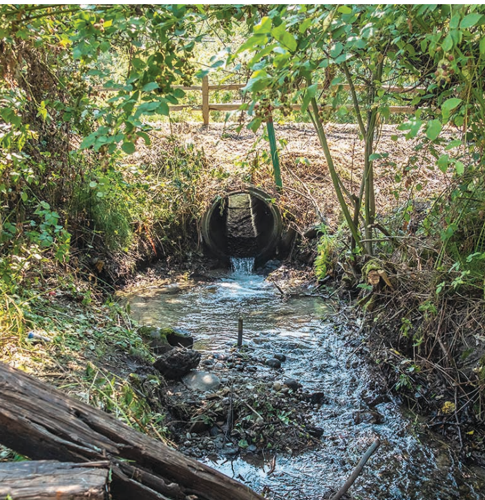
Restoring fish passage, Zackuse Creek culvert replacement (before and after)
