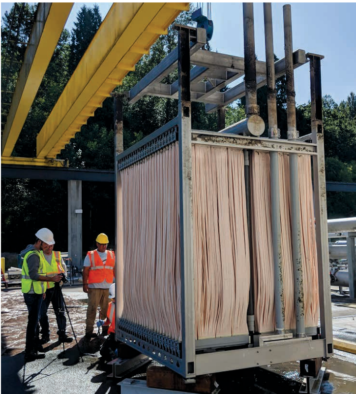
A 2019 upgrade of the “membrane bioreactor” (MBR) at the Brightwater wastewater treatment plant is saving the facility over 2,000,000 kilowatt-hours of electricity each year. The MBR process is a crucial step in creating the high-quality effluent (treated wastewater) produced at Brightwater.
