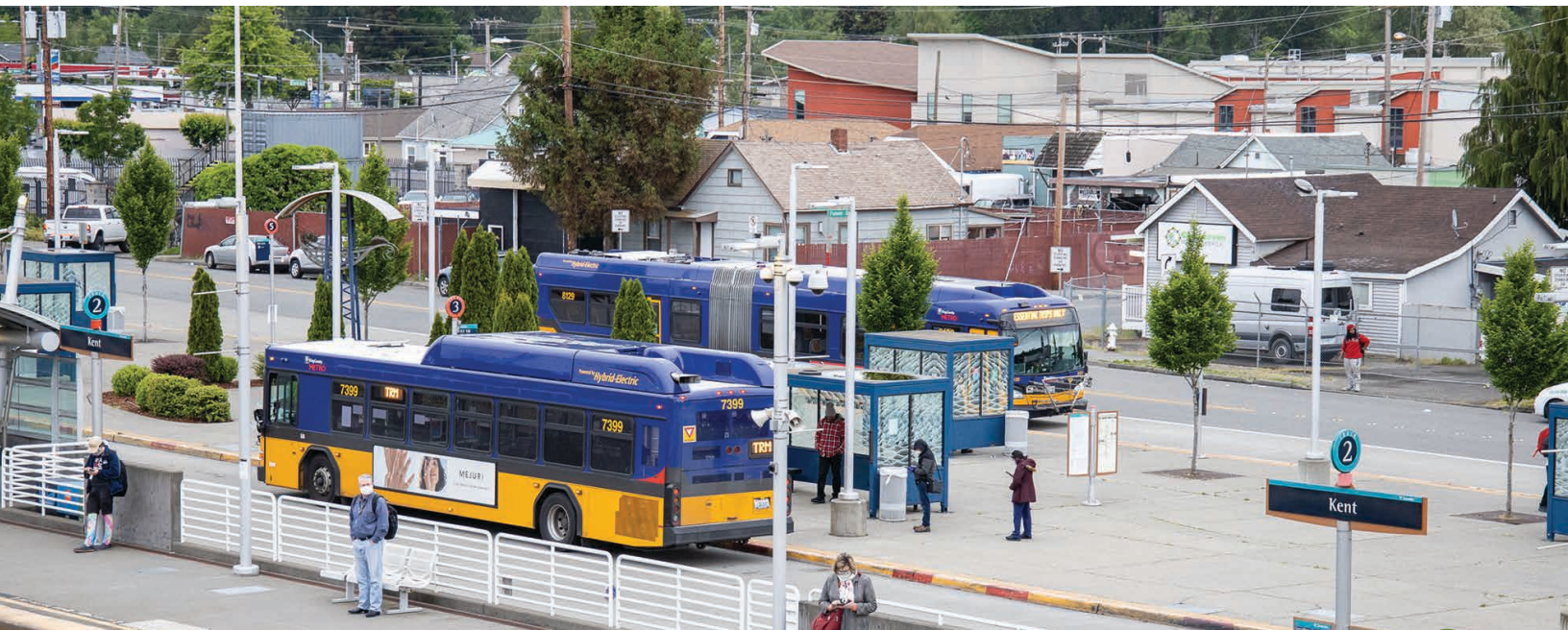
Surrounding area of Kent Transit Center is a regional growth area
