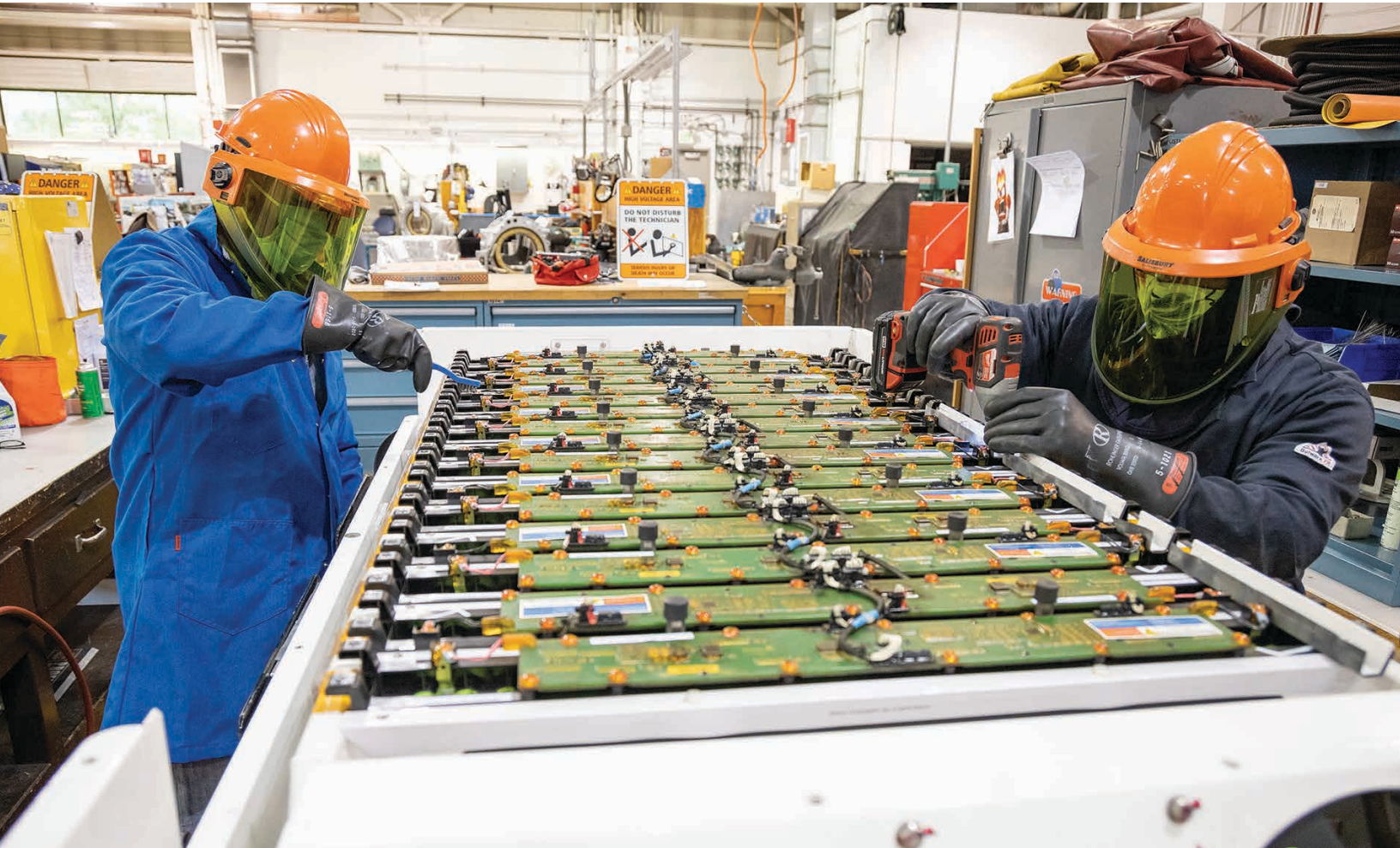
Metro Transit vehicle mechanics replace diesel-hybrid bus batteries.
