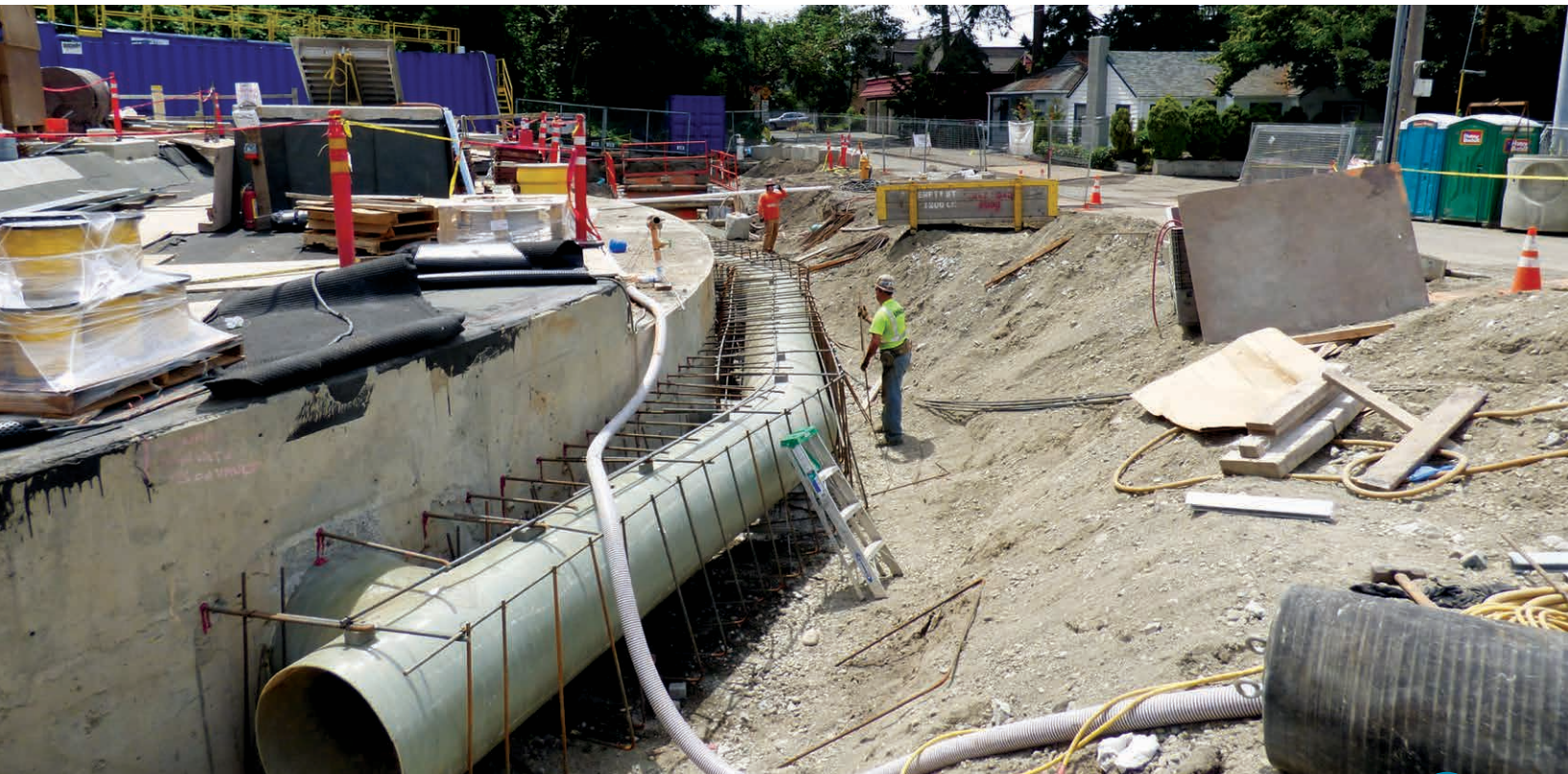
Murray Combined Sewer Overflow Storage Facility construction
