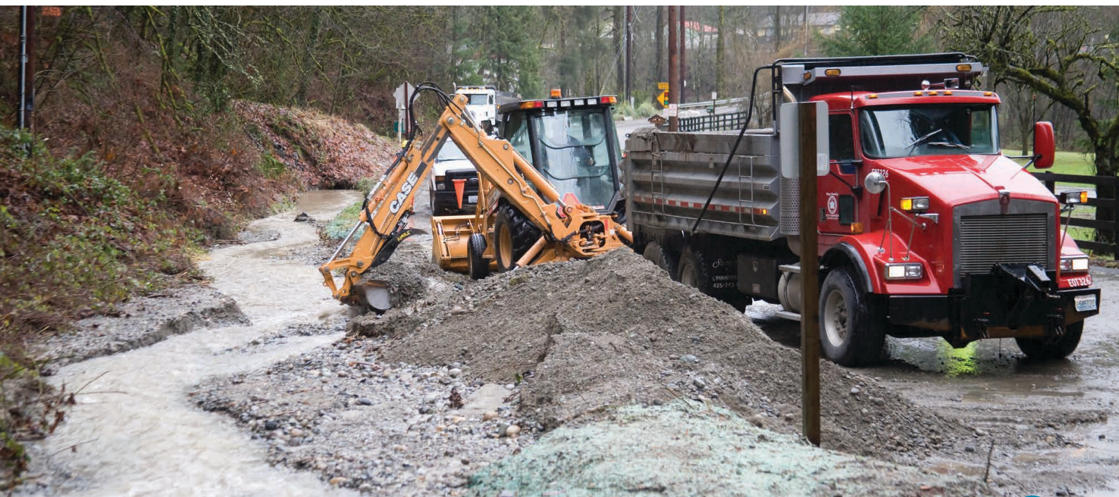
Clearing a landslide from Jones Road (2009)
