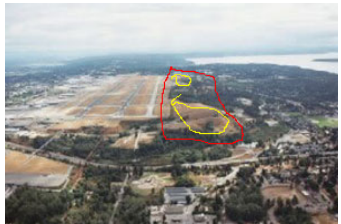
The area outlined in red is the approximate area of the third runway fill. The area outlined in yellow is fill brought in during the past five years—approximately 5 million cubic yards of the eventual 19.84 million cubic yards needed for the runway and an additional 1.13 million cubic yards needed for the Runway Safety Areas.
