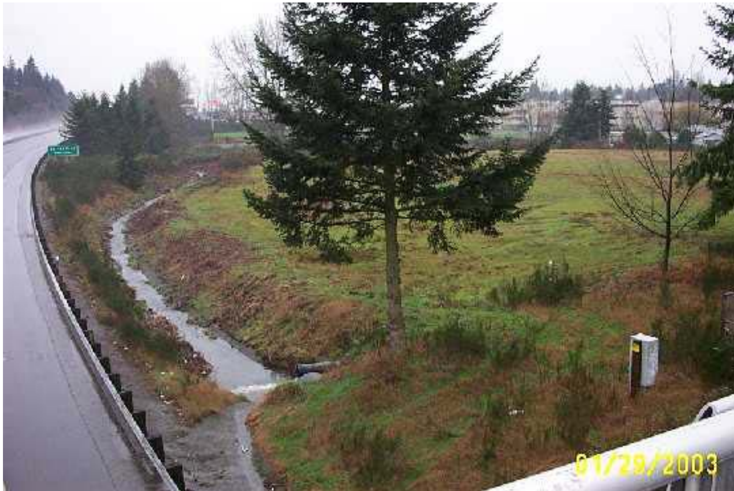
Miller Creek looking south along SR 509 at S. 136 th St.
